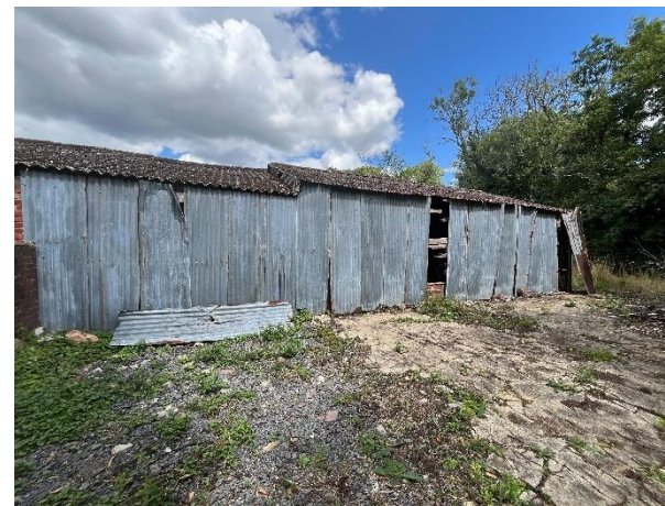
Figure 2. Southern elevation of B1.
