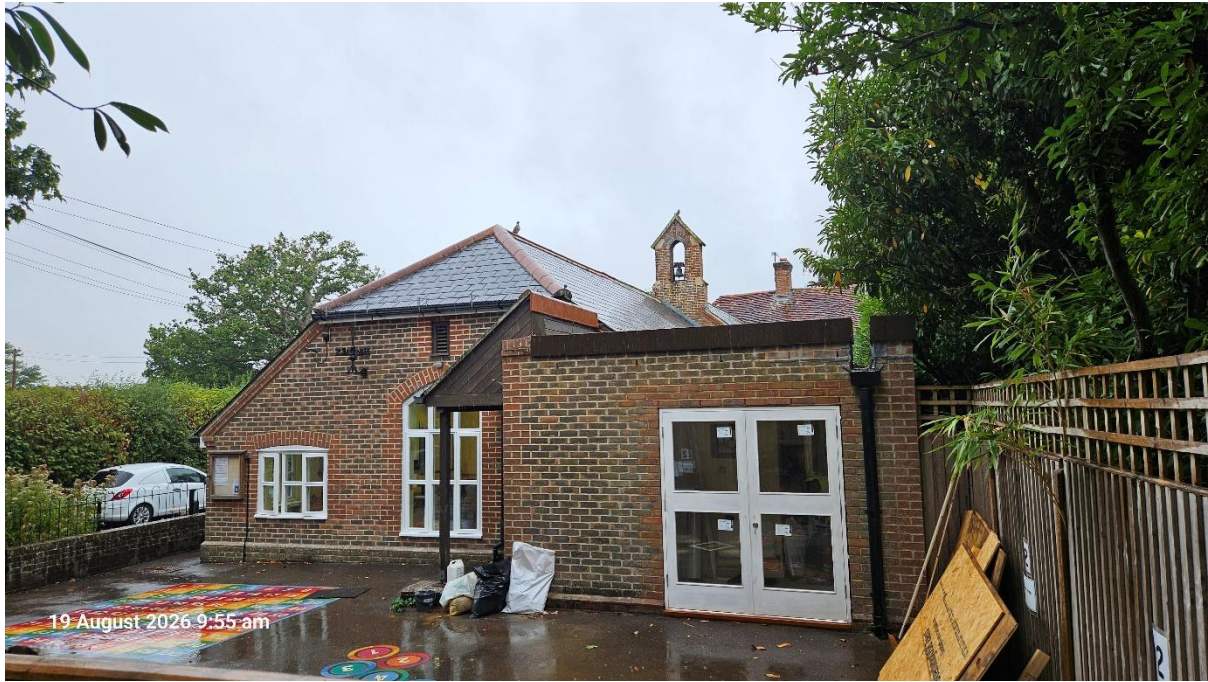
Figure 9 View of school roof from the eastern end of the building. The rear of the school on this side of the building is not accessible due to the fencing abutting the building along the site boundary.
