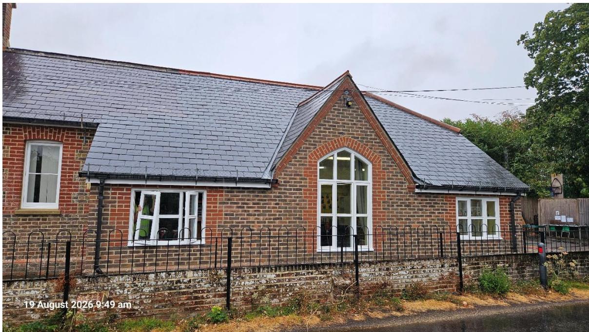
Figure 4 View north from School Lane of the roof where the solar PV panels are proposed to be installed
