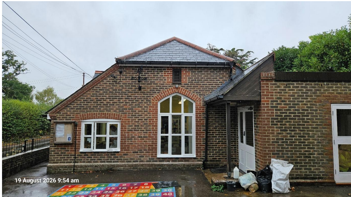
Figure 1 Eastern end of school building, as viewed from the playground
