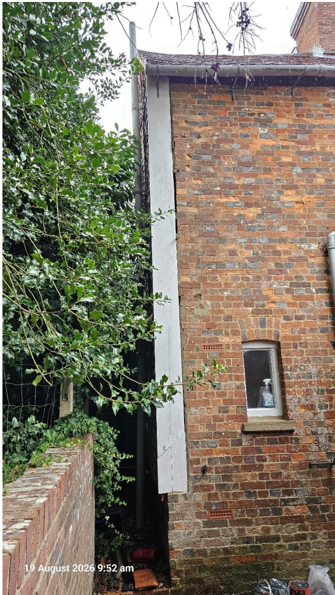
Figure 8 Rear of listed section of school, looking E. Note that access to the rear of the school is limited due to the school building being built up to the edge of the boundary of the site.
