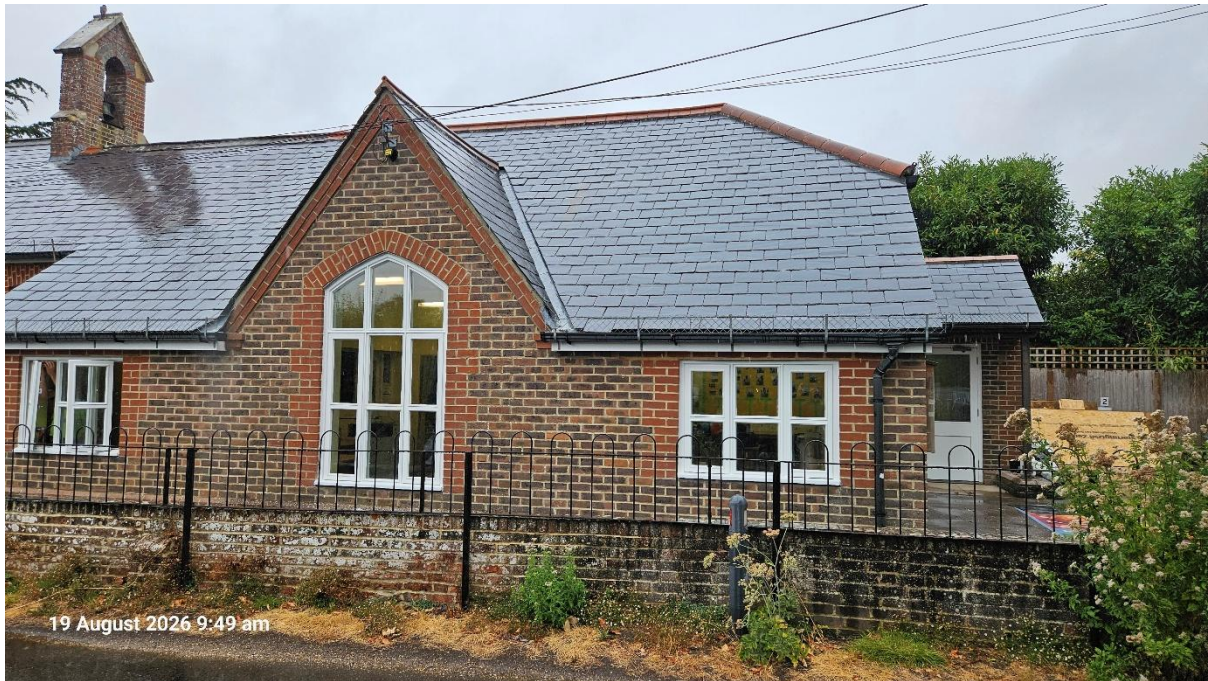
Figure 3 View north from School Lane of the roof where the solar PV panels are proposed to be installed
