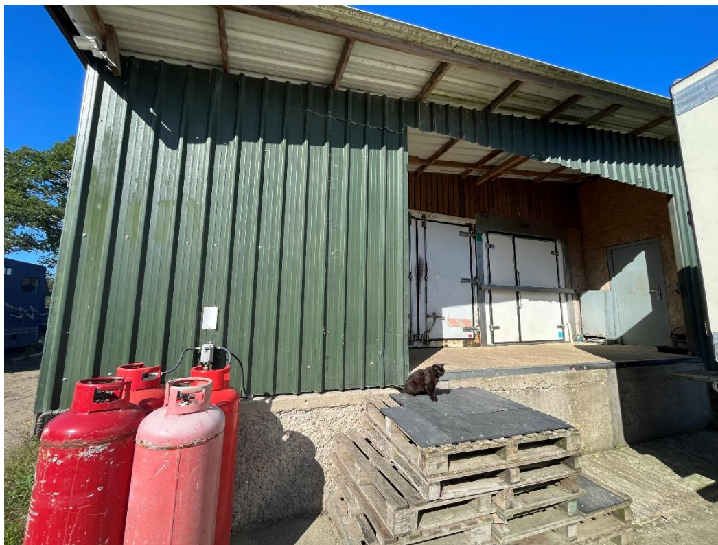
Photo Above: The existing cold store and butchery building to the east of the application building
