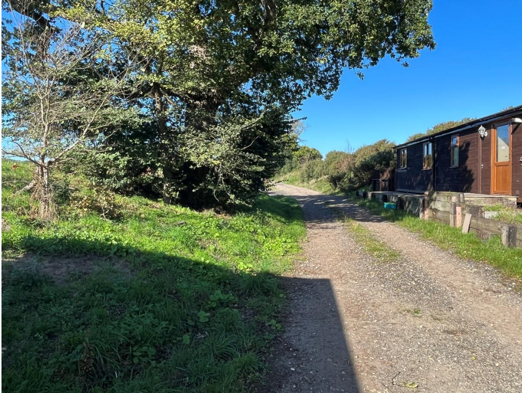
Photo Above: The existing access track and application building
