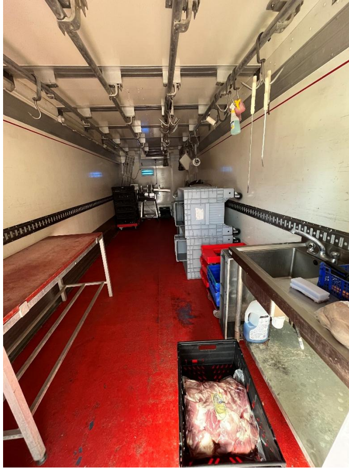
Photo Above: The adjacent cold store and butchery which will be linked to the agricultural training room
