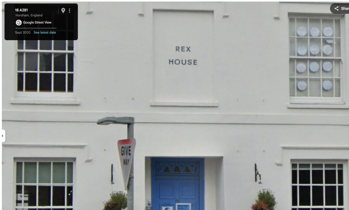
Figure 5: Google Street View image from September 2020 showing visible fixing points in the building
