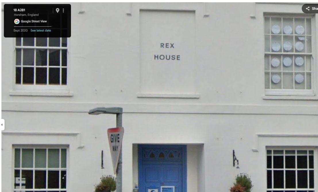
Figure 10: Google Street View image from September 2020 showing visible fixing points in the building
