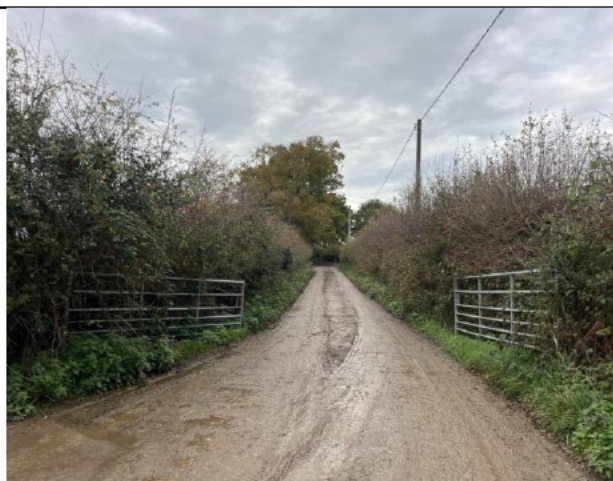
Photograph 6 – Hardstanding access track connecting the development area to the main road.
