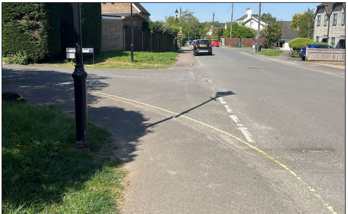
Figure 3.7: Footways Along Rectory Lane (Looking West at Windmill Close)
