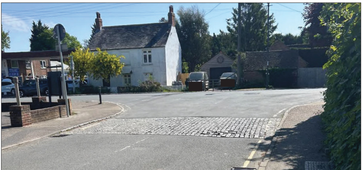
Figure 3.16: Tactile Paving and Dropped kerb at Rectory Lane/London Road junction
