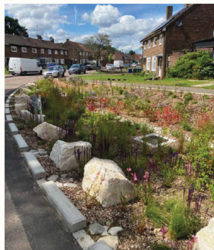
Rain garden integrated into verge alongside residential street
