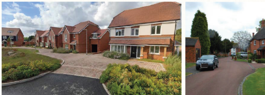
Examples of surface changes as a traffic calming measures - on shared surface and junctions
