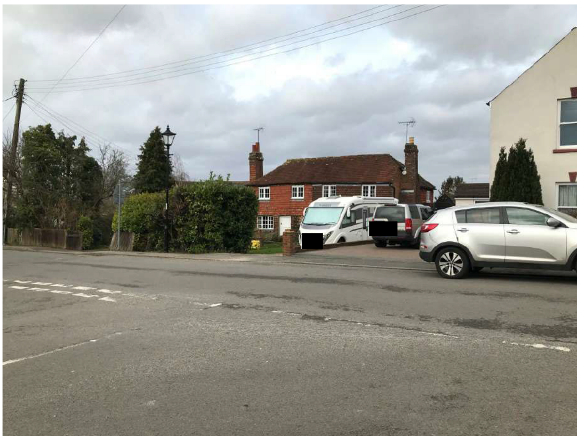
Plate 12: View of Laurel and Orchard Cottage from south side of Rectory Lane, looking north west.
