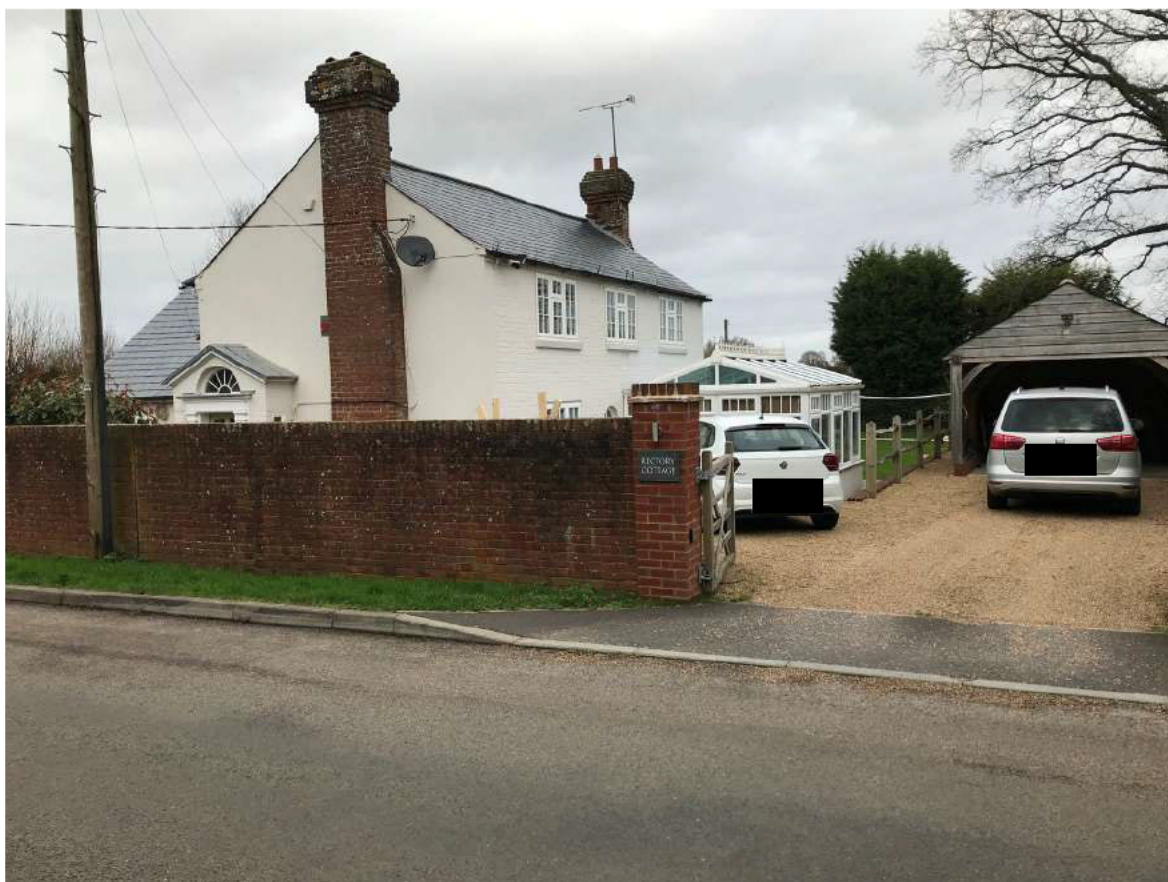
Plate 7: Rectory Cottage as seen from Rectory Lane, looking north-north west.
