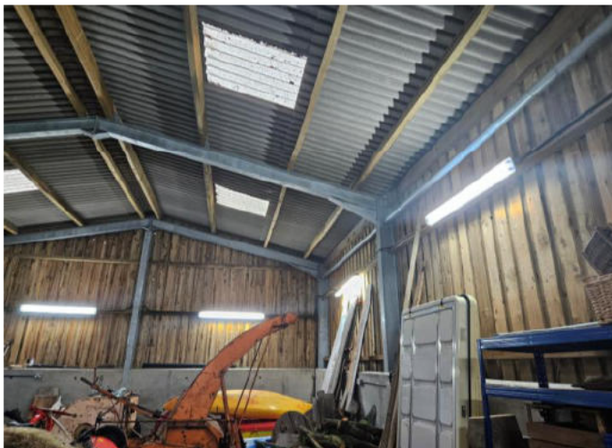
Photo 5: Displaying gaps between timber cladding on the southeastern aspect of building B1 within the development boundary.
