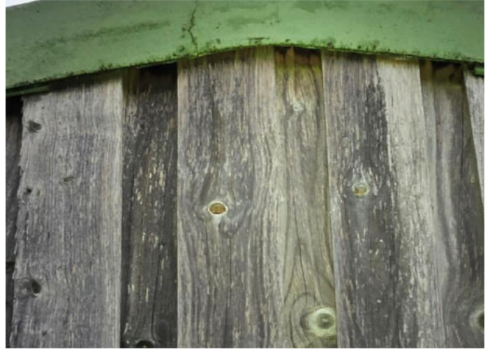
Photo 6: Displaying gaps in timber providing access to the interior of building B1 within the development boundary.
