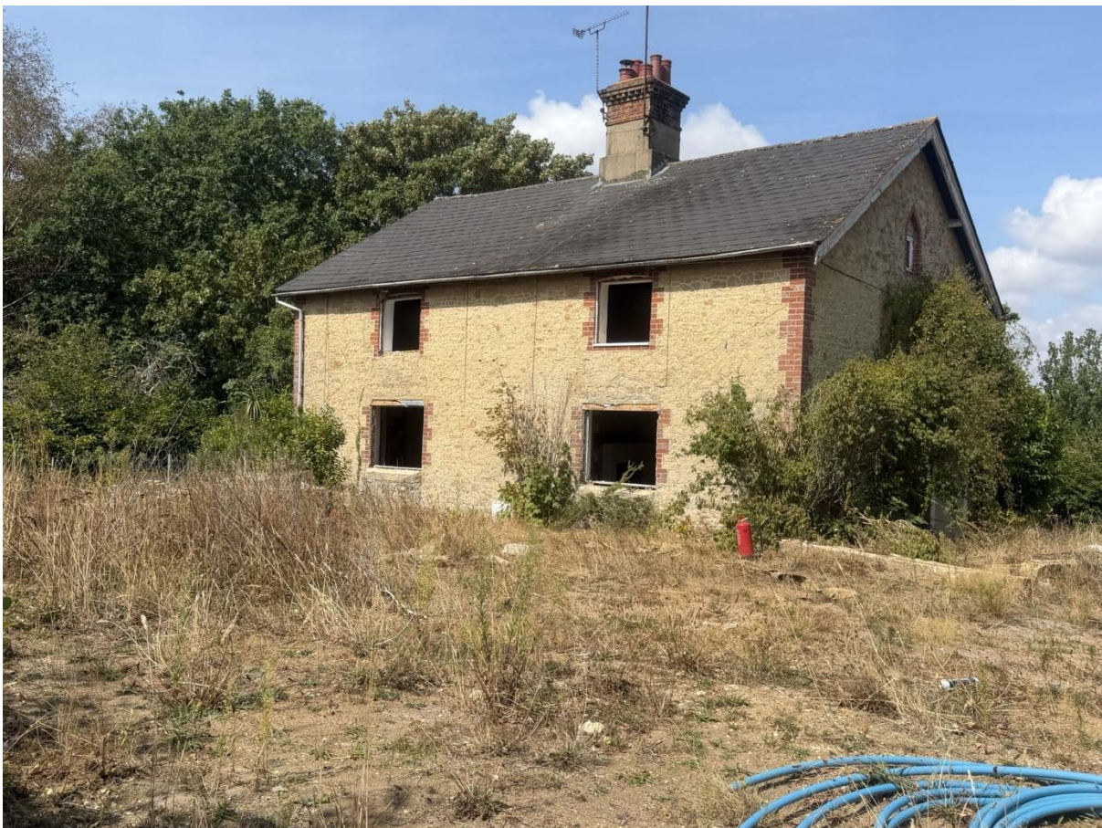
Threals Farm Cottages as viewed from the south eastern corner of the Site. A pair of semi-detached farm workers cottages with the white upvc windows removed. (2026)
