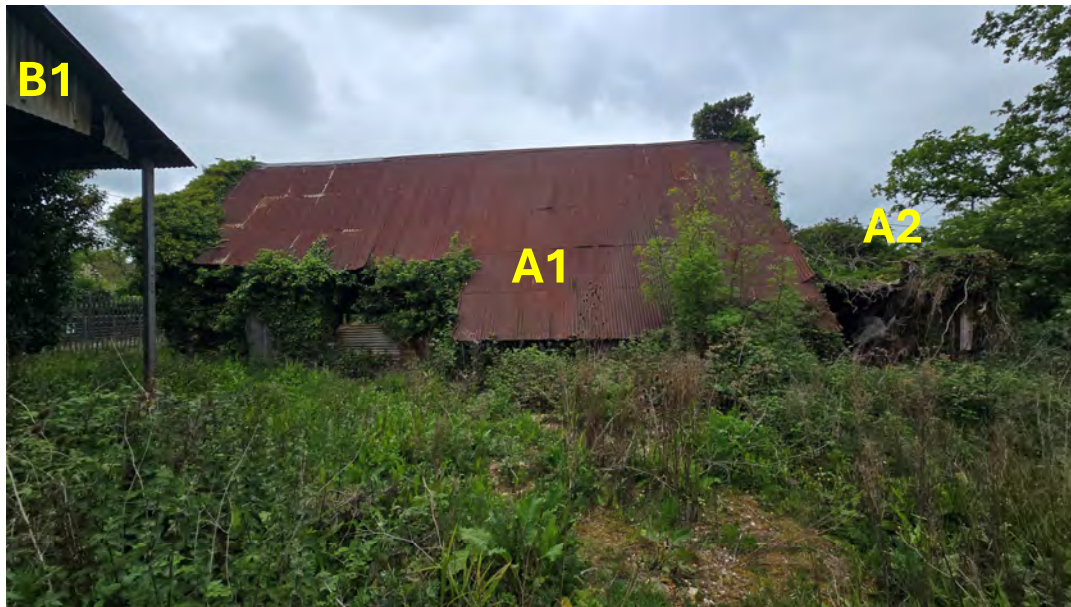
Figure 3. Shows the Sussex Barn from inside the subject site with the A2 Attached Hovel.
