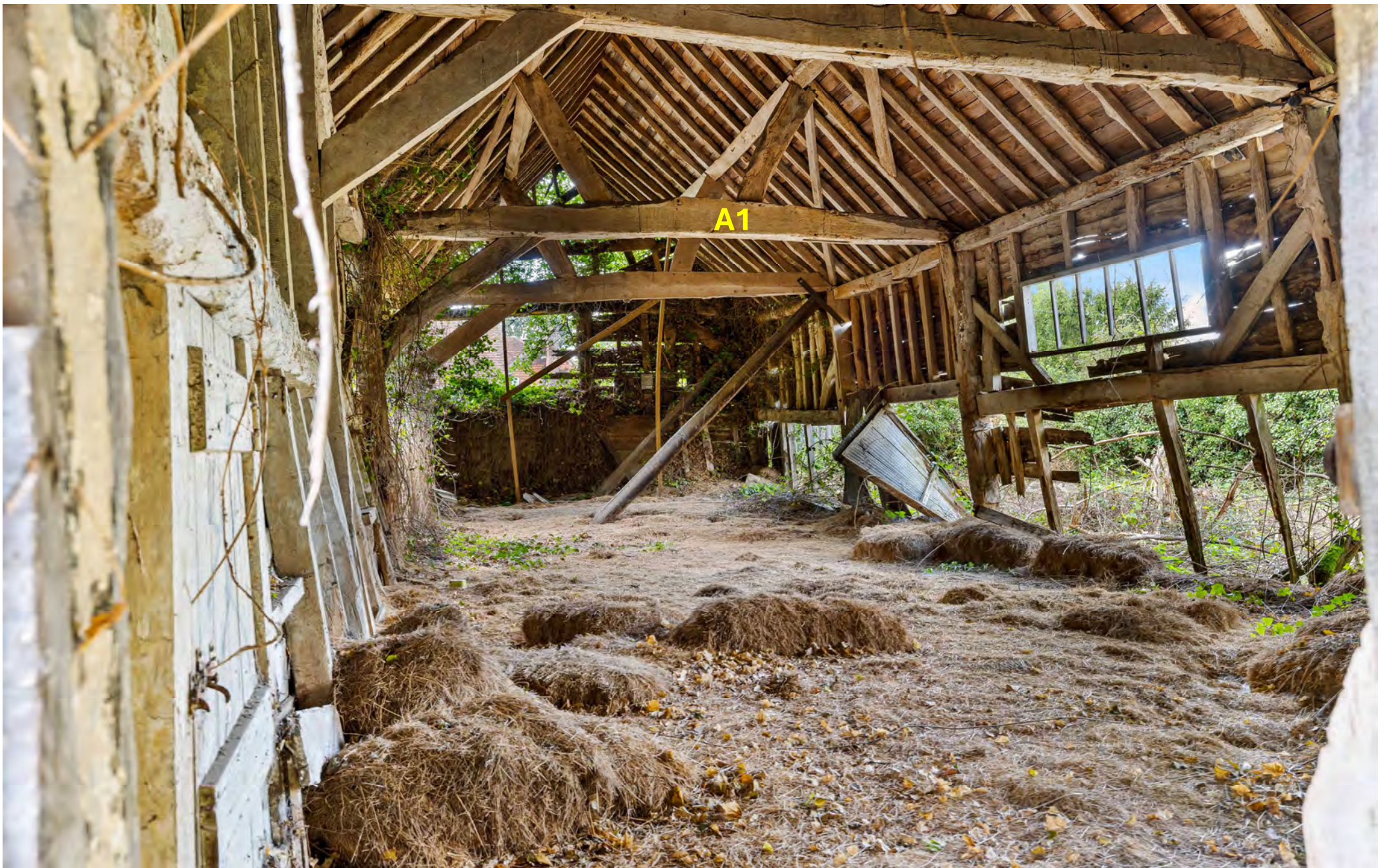
Figure 15. Inside The Sussex Barn June 2024 (photos used for marketing)
