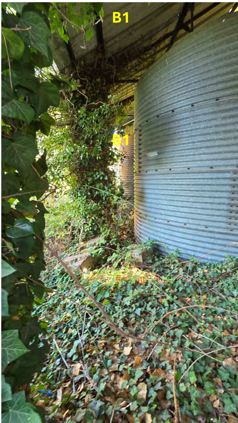
Figure 8. View within B1 showing the two corrugated grain silos beneath the raised roof structure.
