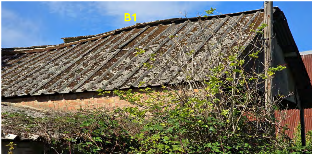
Figure 7. Closer view of B1 showing its raised roof form and brick flank wall above the adjoining lower roofed range.
