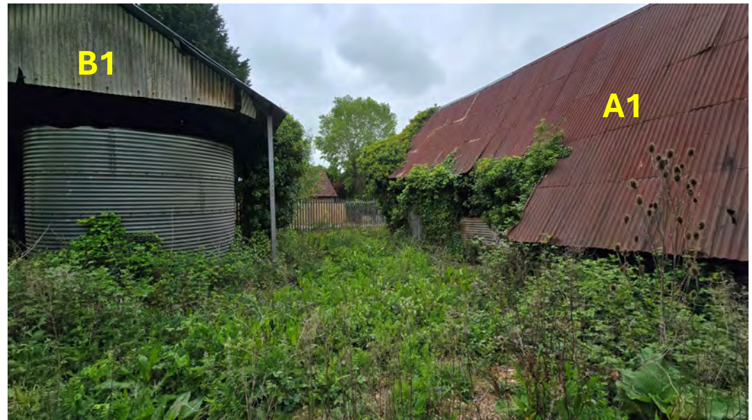
Figure 4. Shows both the Sussex Barn and B1 Western end silo bay to the left.
