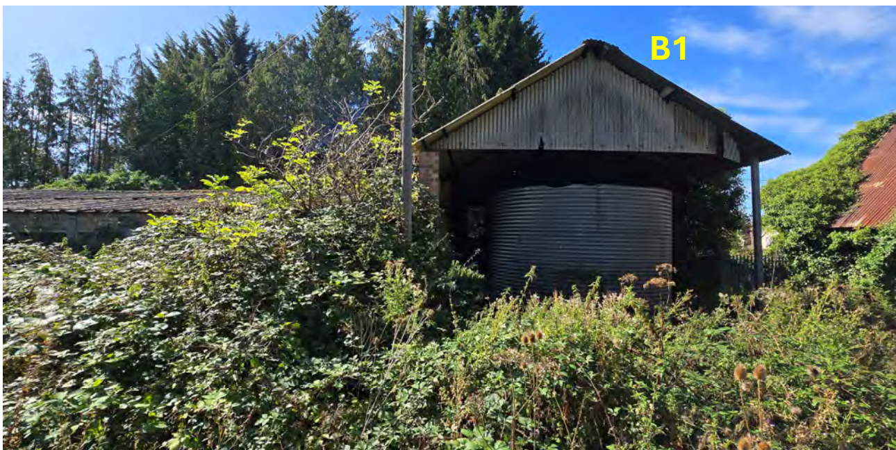
Figure 10. View of B1 showing the raised western end silo bay and the change in height and roof form relative to the adjoining lower range.
