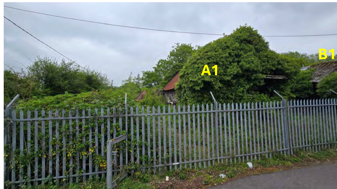
Figure 2. Sussex Barn viewed from driveway beyond fence.
