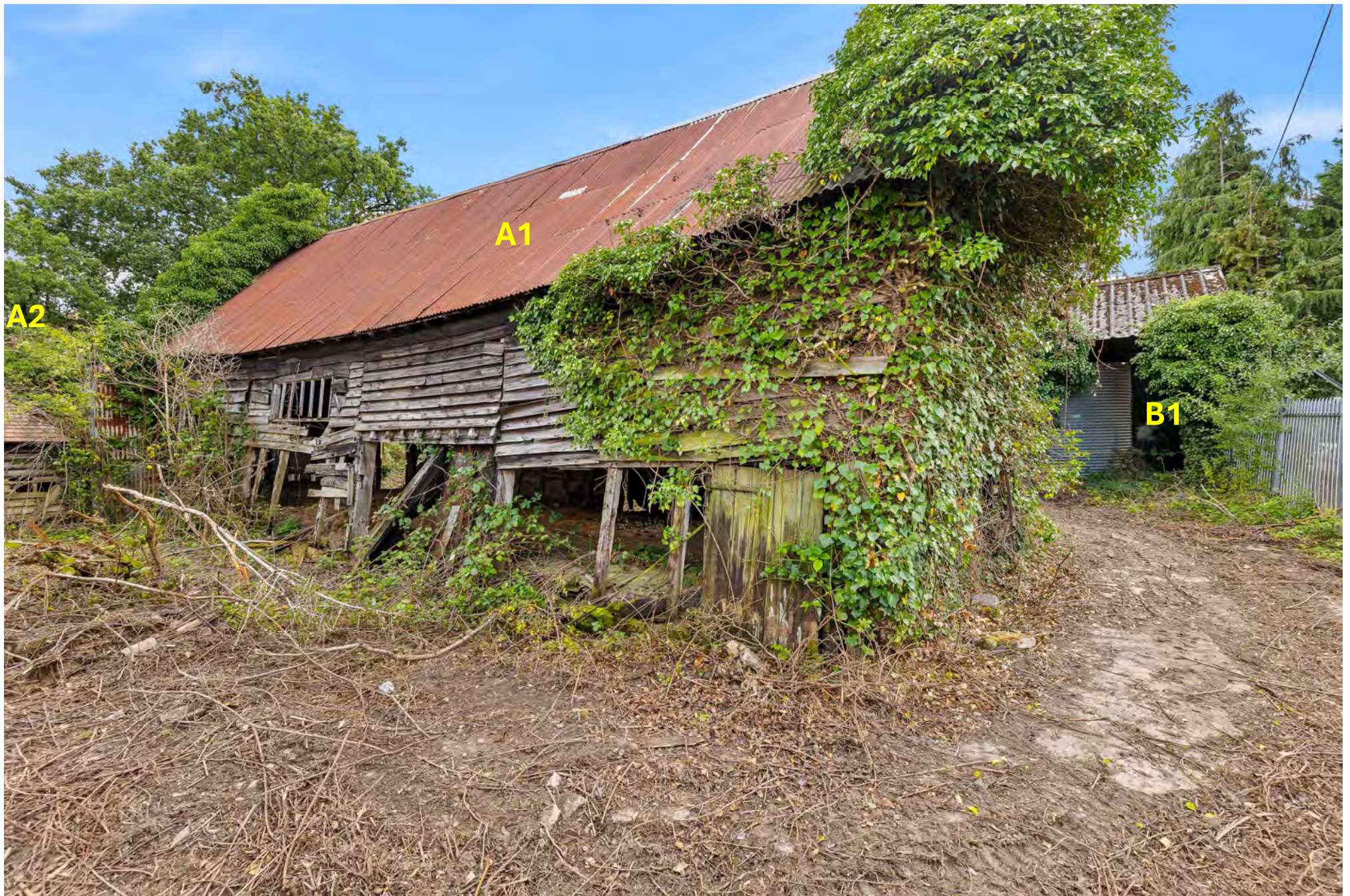
Figure 16. View showing the Traditional Sussex Barn centrally, the western end Silo Bay to the right and the attached Hovel to the left, following vegetation clearance in June 2024.(photos used for marketing)
