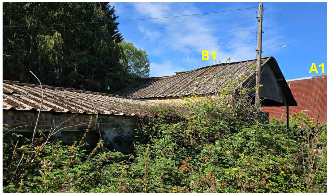
Figure 6. View of B1 from the east, showing the distinct raised western end silo bay in relation to the adjoining lower roofed range and the Traditional Sussex Barn (A1)
