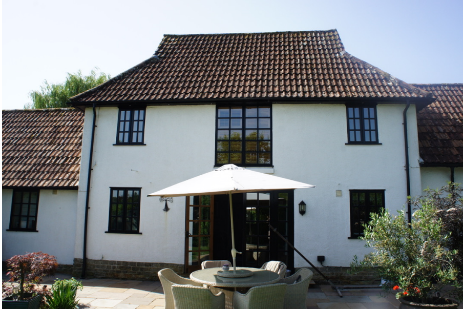
Figure 1 – Rear (principal garden) elevation of 3 The Old Sussex Stud illustrating the simple architectural form, uninterrupted clay pantile roofscape and restrained architectural detailing.
