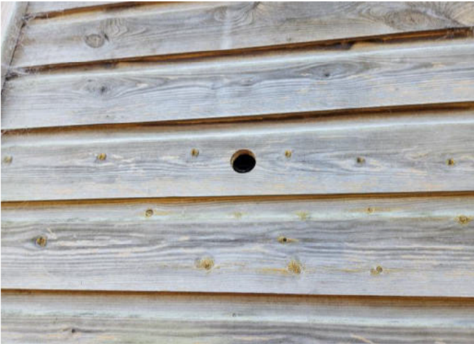
Photo 5: Displaying a hole in wooden cladding on the northern elevation of building B1 within the development boundary.
