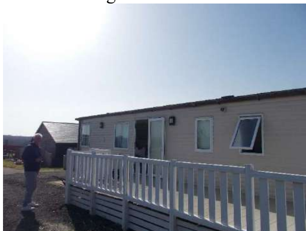
Existing caravan to the east
