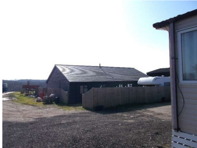
Existing eastern building to be retained
