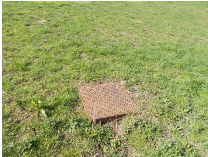
Existing manhole leading from sewage treatment plant
