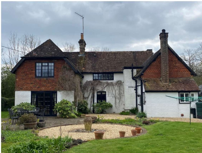
Photograph showing the rear of the property. Original House and kitchen outshot to the right of the photograph, 1900 section in the centre, 1970s section to the left of the photo
