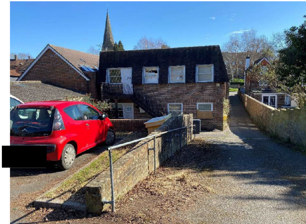
Figure 3 - Photograph of the Rear (West) Elevation showing the rear façade of the building and part of the car park to the rear of the site
