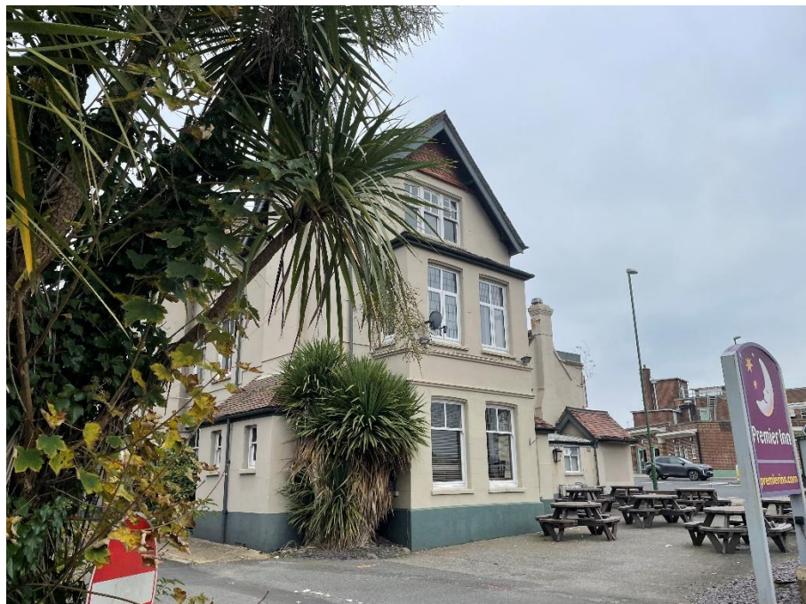
The restaurant (looking northeast from Hurst Road)
