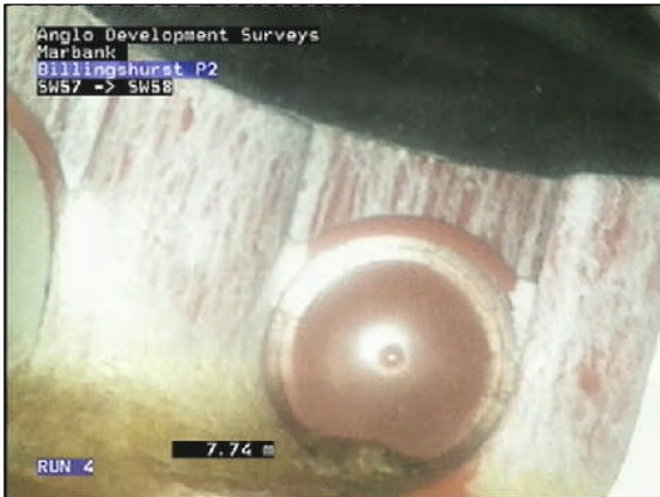
Photo: 5_5_15_A.JPG 7.7m, Finish node type, manhole reference number: SW58
