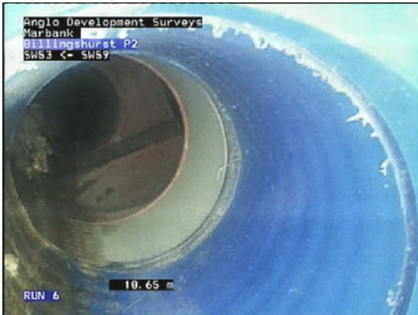
Photo: 7_7_22_A.JPG 10.6m, Finish node type, manhole reference number: SW59
