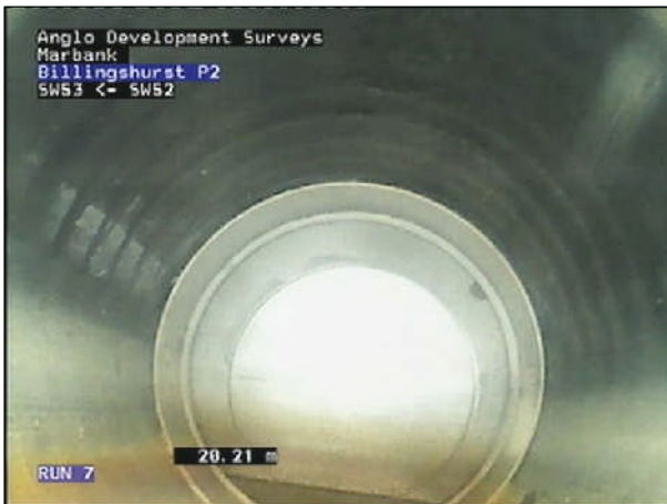
Photo: 8_8_25_A.JPG 20.2m, Finish node type, catchpit reference number: SW52
