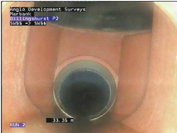
Photo: 3_3_8_A.JPG 33.3m, Finish node type, manhole reference number: SW56
