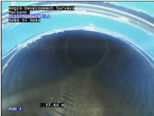
Photo: 1_1_5_A.JPG 17.6m, Finish node type, manhole reference number: SW54
