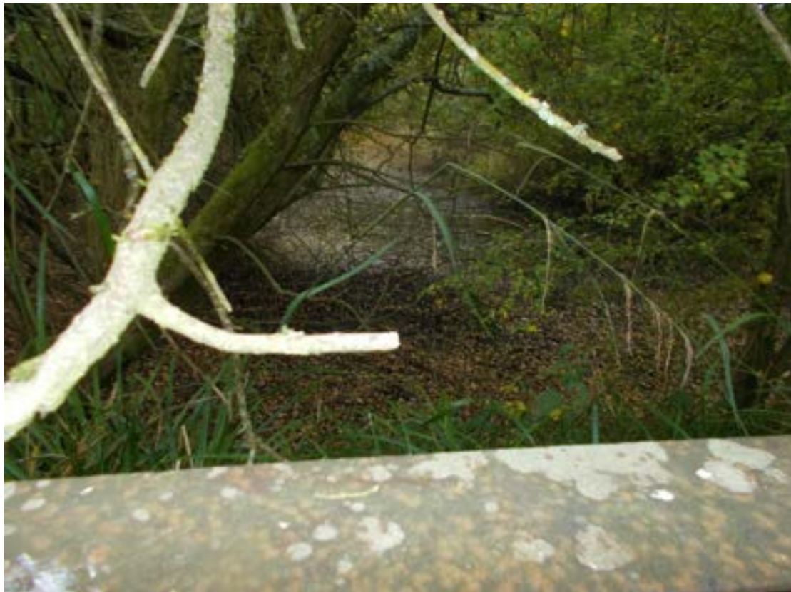
Flooded and overgrown sileage (never used)
