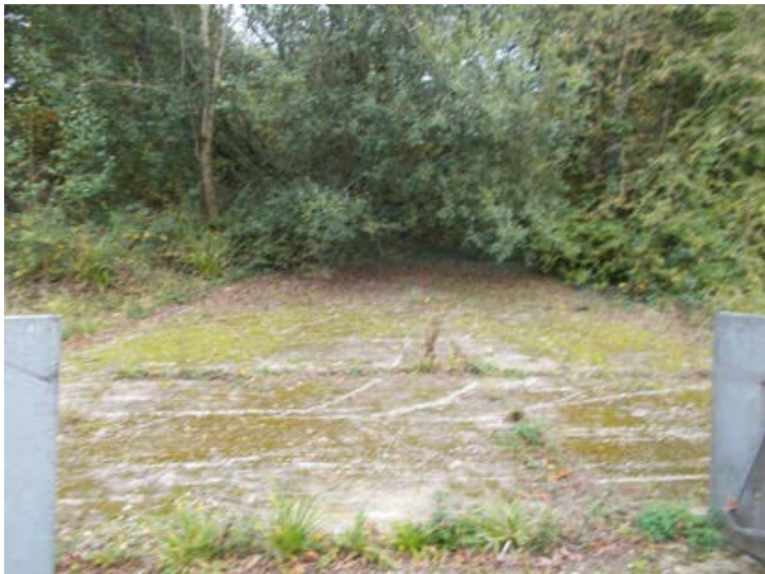
Ramp rear of Barn D
