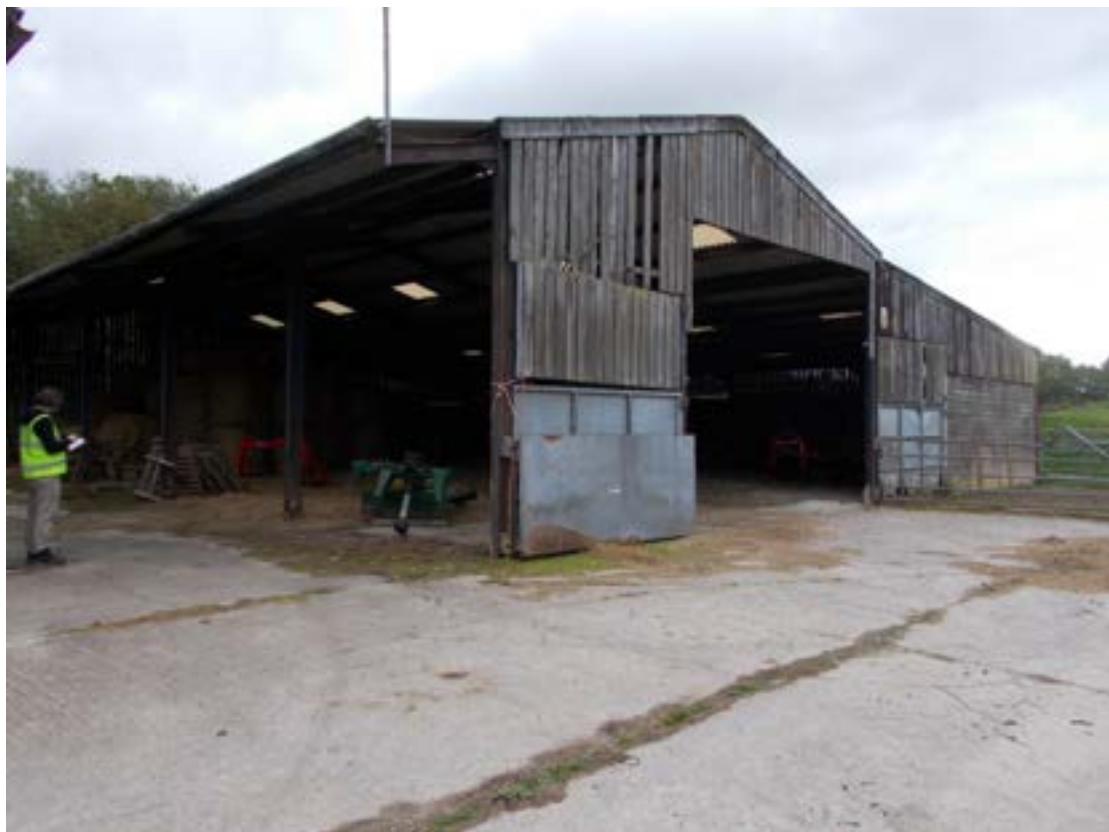
Barn E Northern and eastern façades
