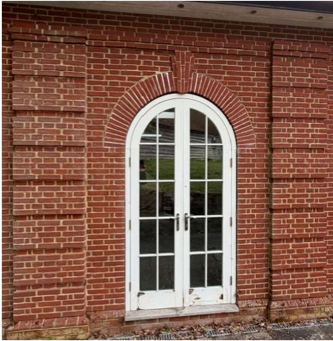
Brick detailing of 2007 Orangerie extension based on original ballroom with hardwood timber French doors. This opening is 1.2m versus the proposed at 2m
