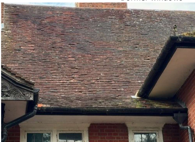
Sprung eaves where the roof pitch shallows as it approaches the gutters
