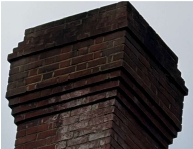
Chimney stack brickwork detail
