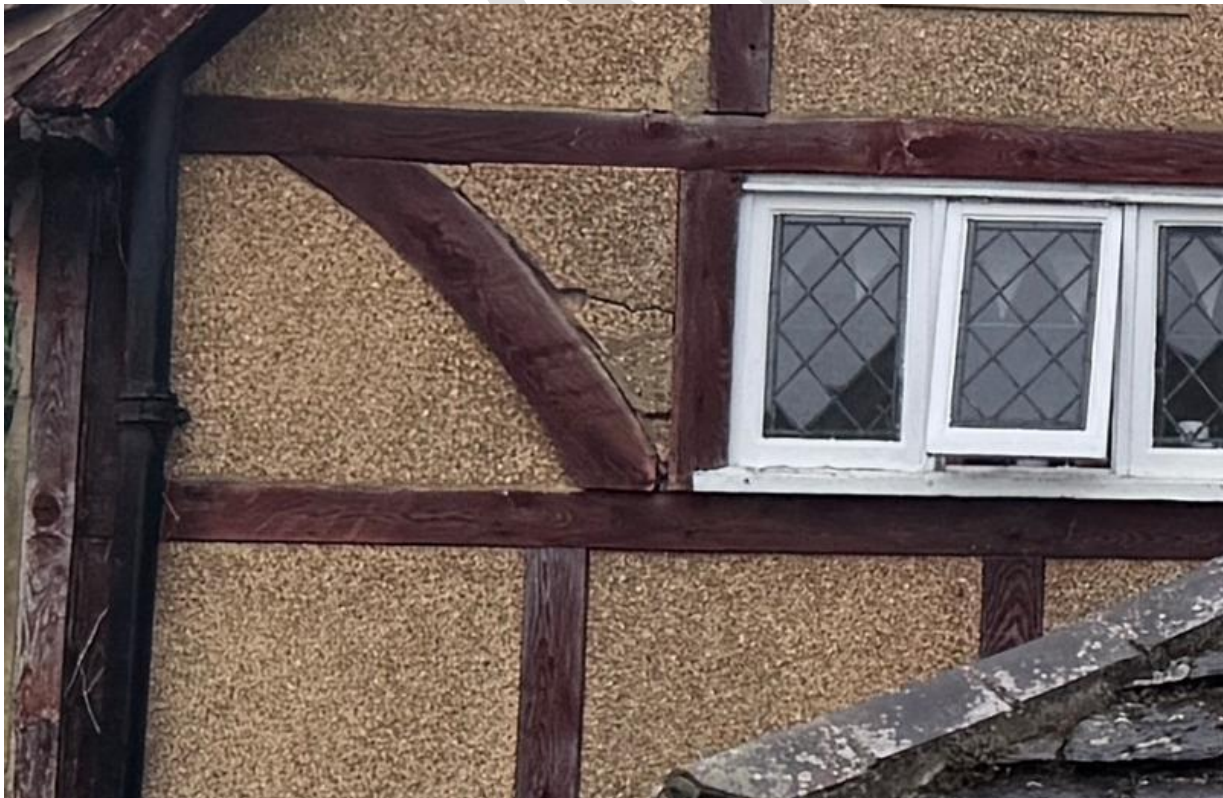
External note 3 – Spalled pebbledash render between timbers
