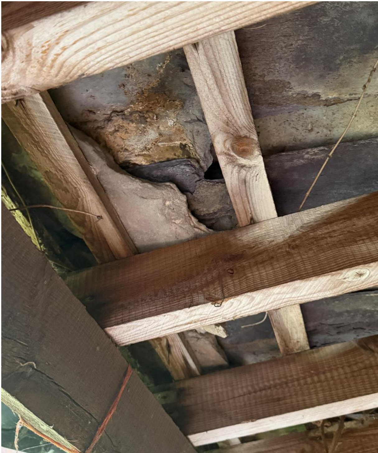
External note 7 – view beneath shelter running length of north east aspect illustrating roof tile detail
