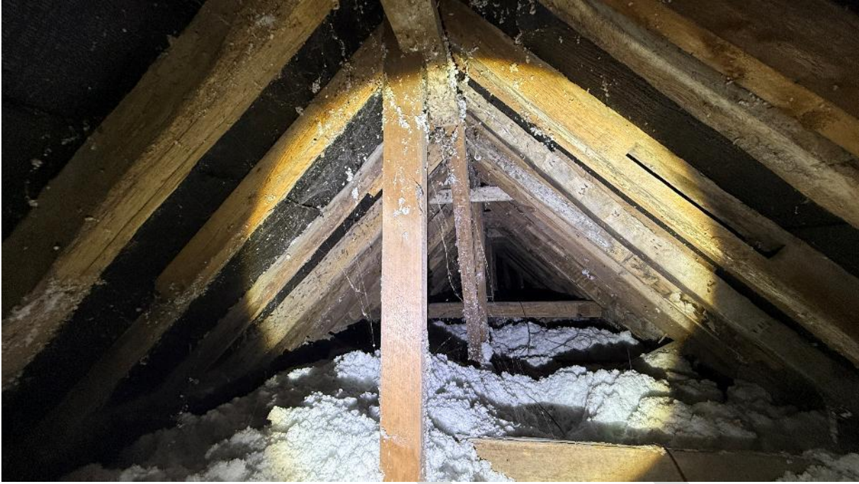
Internal note 1 – king post roof showing blown-in insulation
