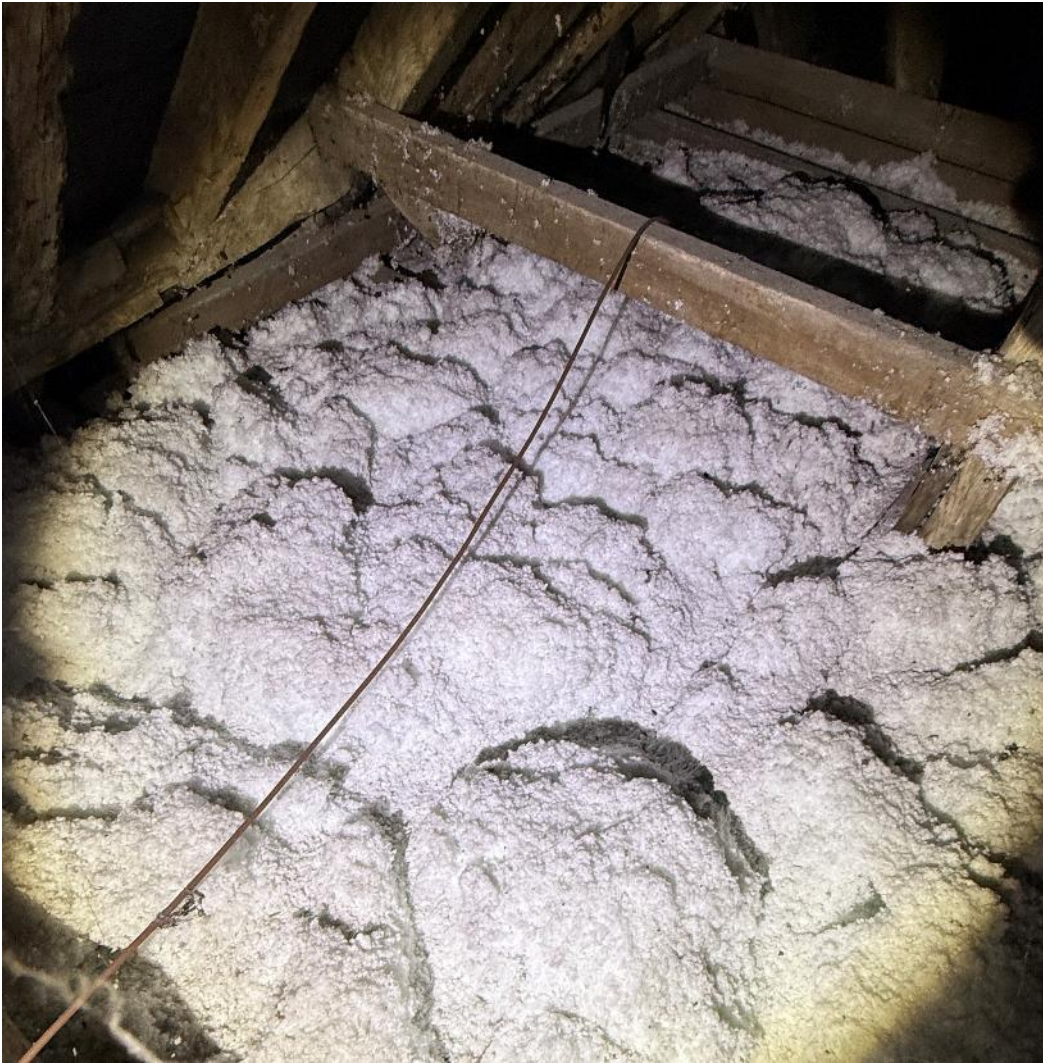
Internal note 1 –blown-in insulation with extensive rodent runs and droppings
