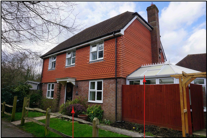
Existing principal Elevation and conservatory
