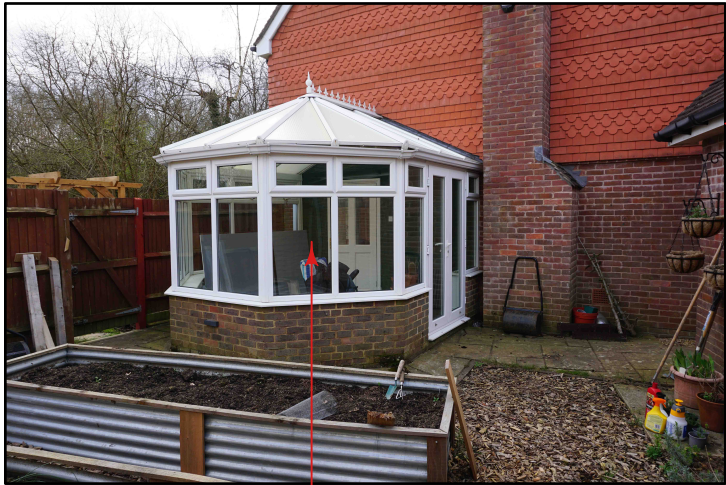
Existing conservatory to be replaced
