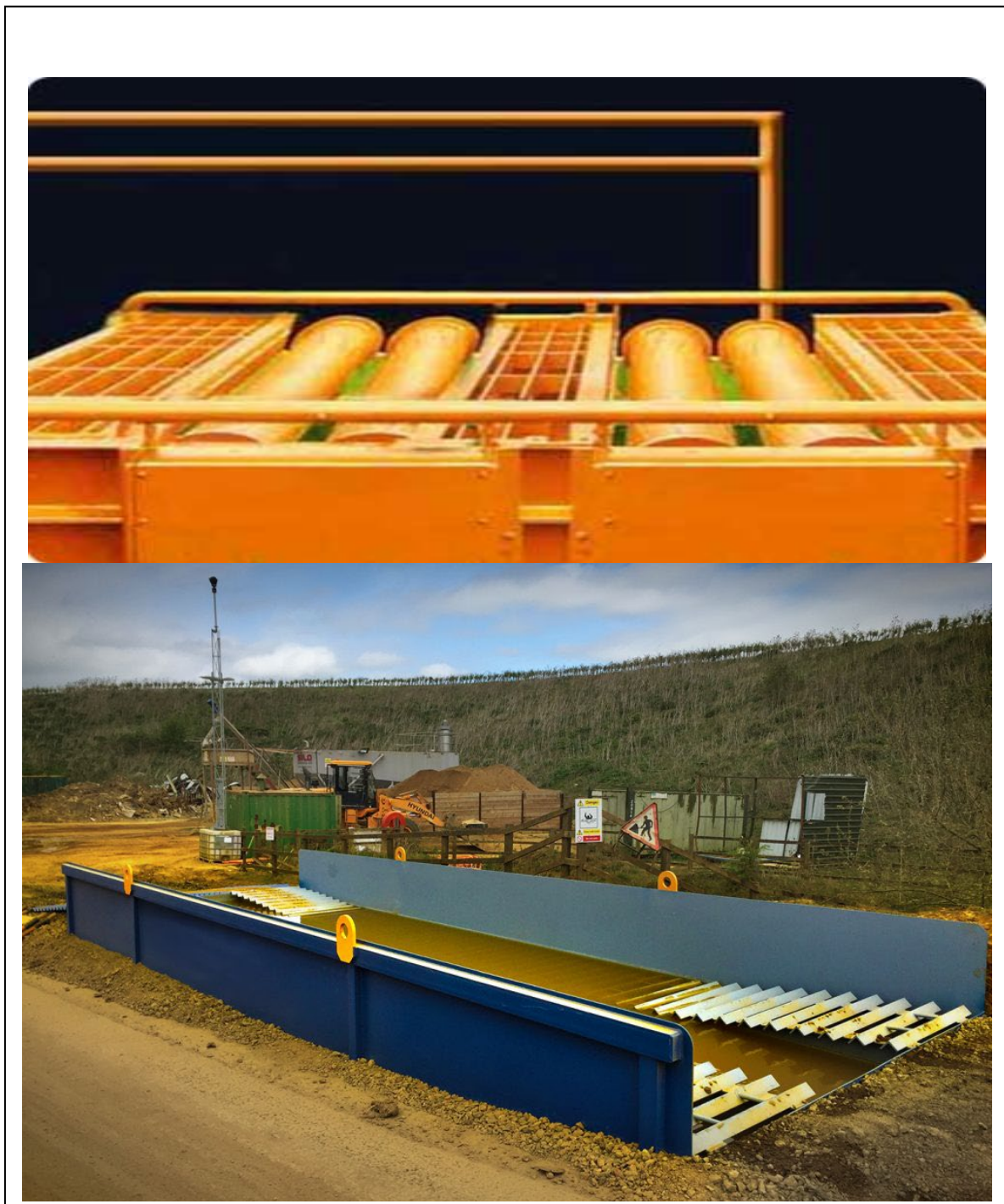
Example of wheel cleaning facility
