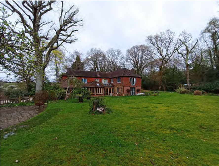
Existing Main house
