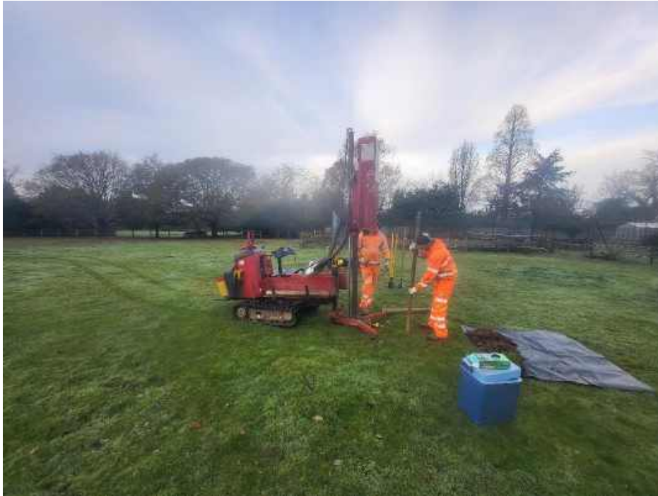
Photo 3 - Tracked window sampler at BH2
