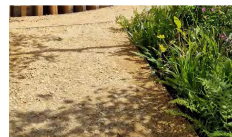
Self Binding Gravel path in the POS
