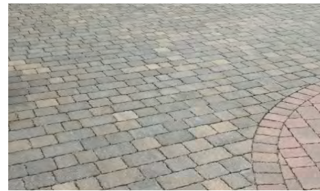
Non permeable Block Paving for Access Road
