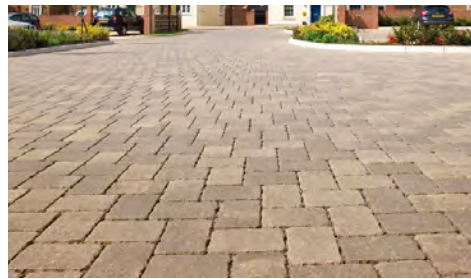
Permeable Block Paving
