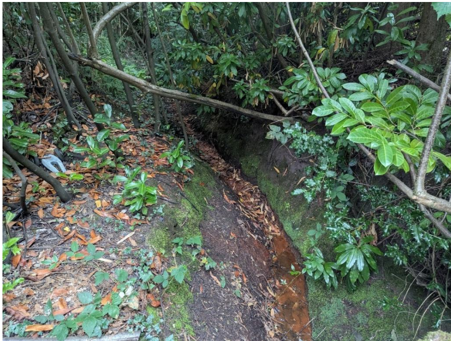
Figure 5. Ditch present on site (taken August 2025).
