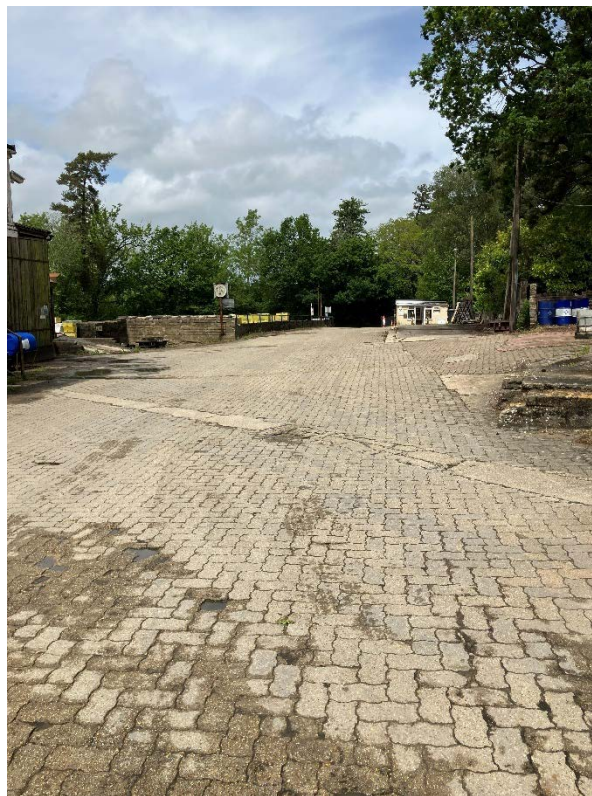
Photograph 64: Northern part of site – towards site entrance, weighbridge and reception. Looking north.
