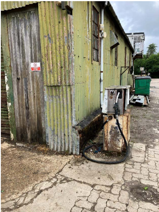
Photograph 40: Disused fuel pump. Looking north.
