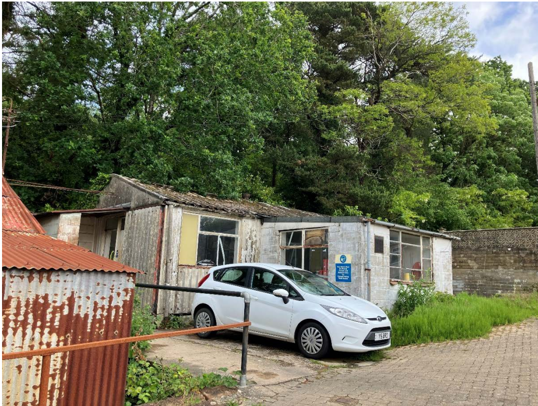
Photograph 59: Canteen building in northeastern area of site. Looking northeast.
