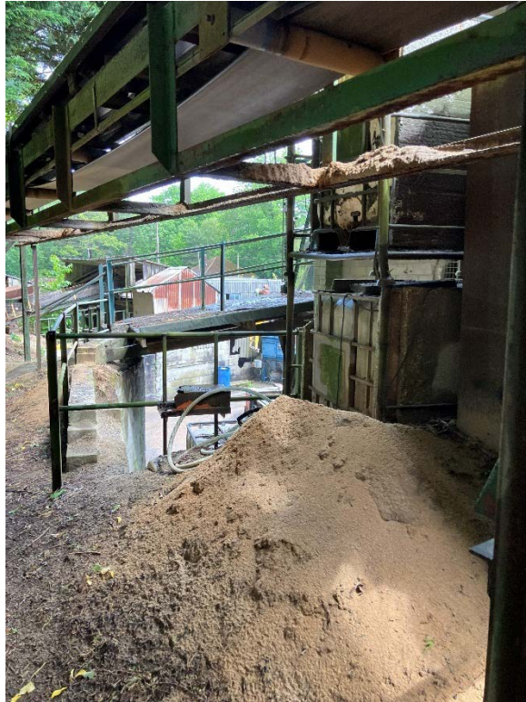
Photograph 33: Conveyor infrastructure close to western site boundary. Looking north.
