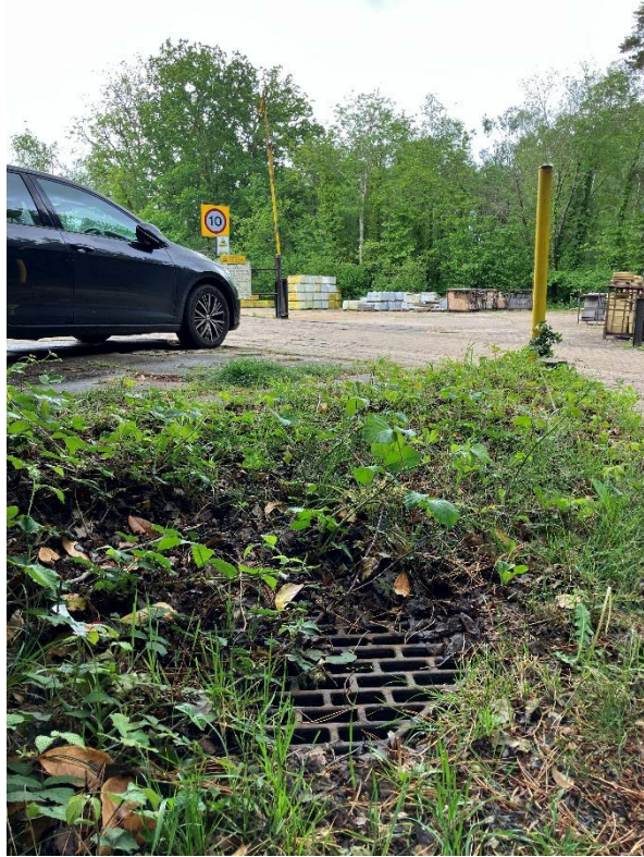
Photograph 55: Drainage along northern boundary at site entrance from Rock Road.
