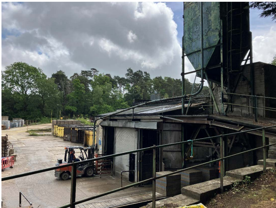
Photograph 35: Building assigned to manufacture of blocks. Looking southeast.
