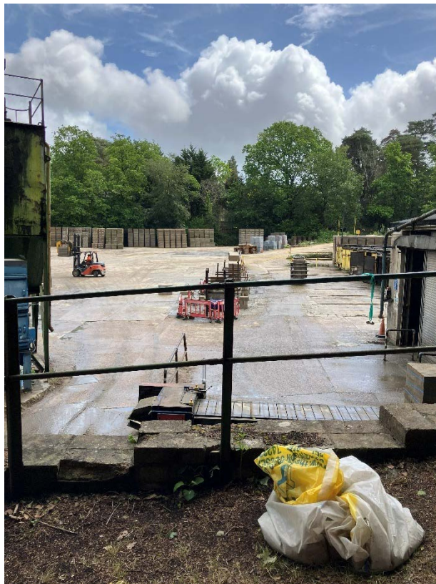
Photograph 34: Overview of central area of site – manufacture, curing and storage of blocks, pavers. Looking east.
