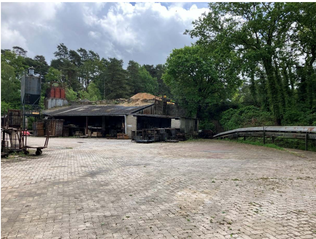
Photograph 30: Building and storage areas, with conveyor, in central area of site. Looking southeast.
