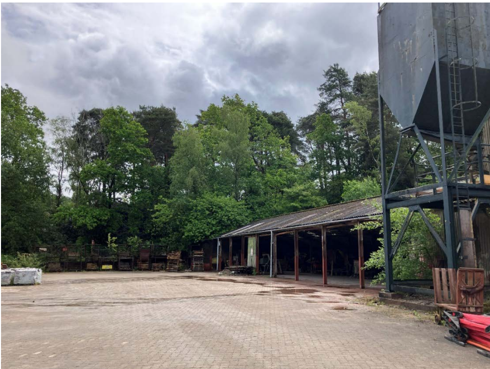
Photograph 4: Storage areas (pallets at far end) with historical processing infrastructure. Looking east.
