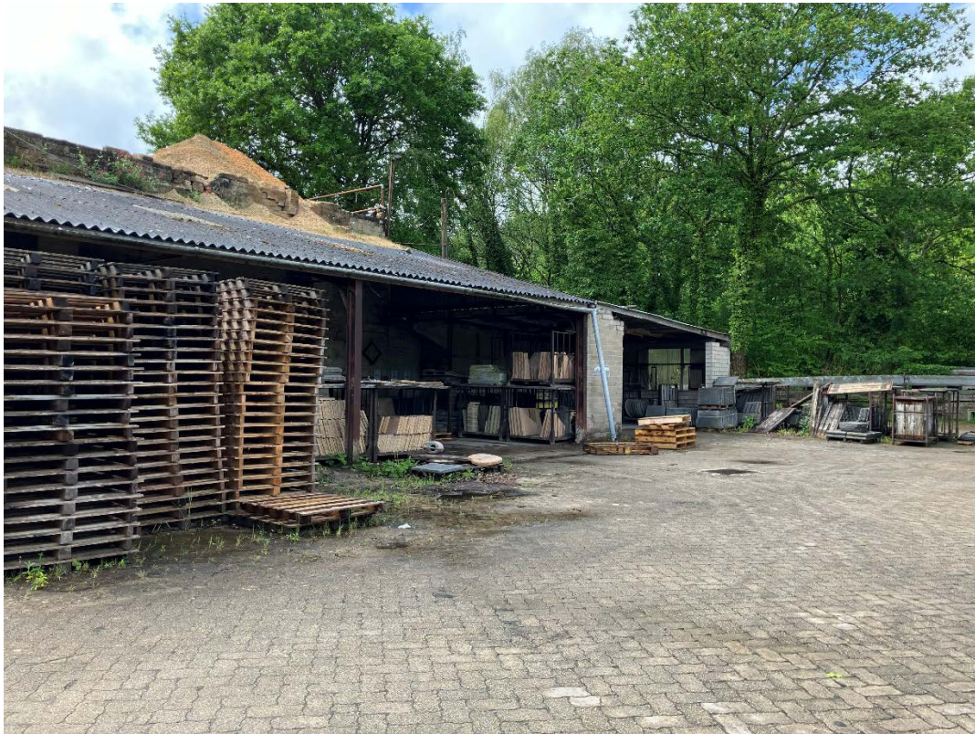
Photograph 5: Storage of manufactured paving slabs. Looking west.
