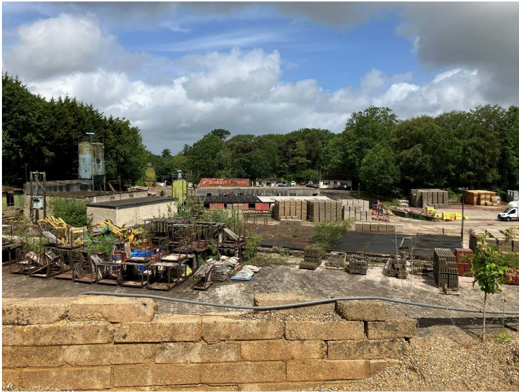
Photograph 25: Overview of site from materials storage area in south. Looking north.
