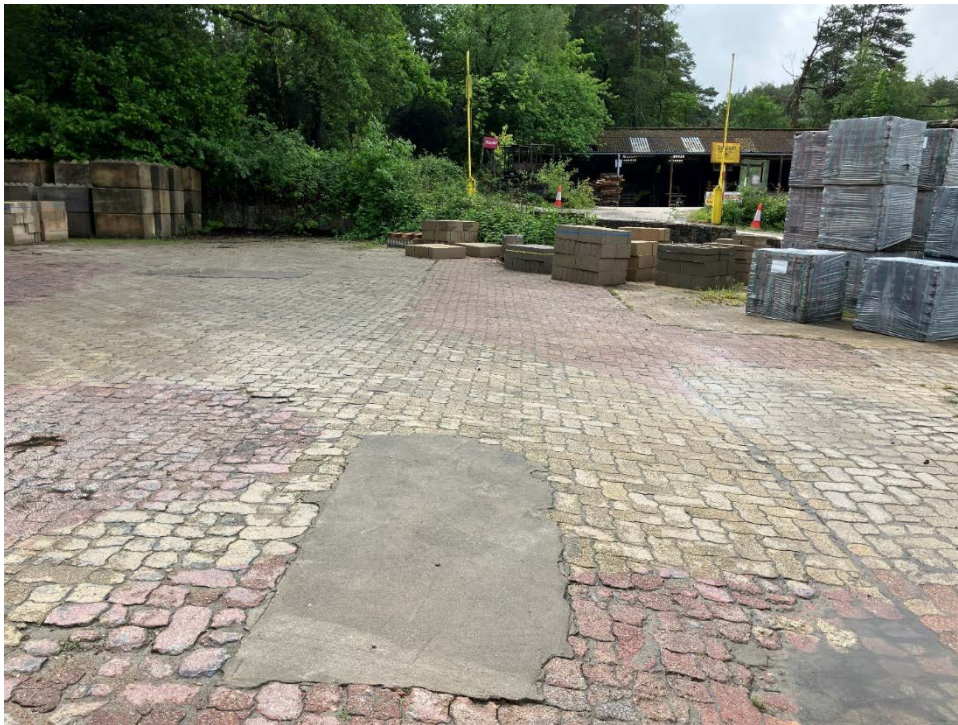
Photograph 3: Evidence of previous ground investigation in central east part of site. Looking south.
