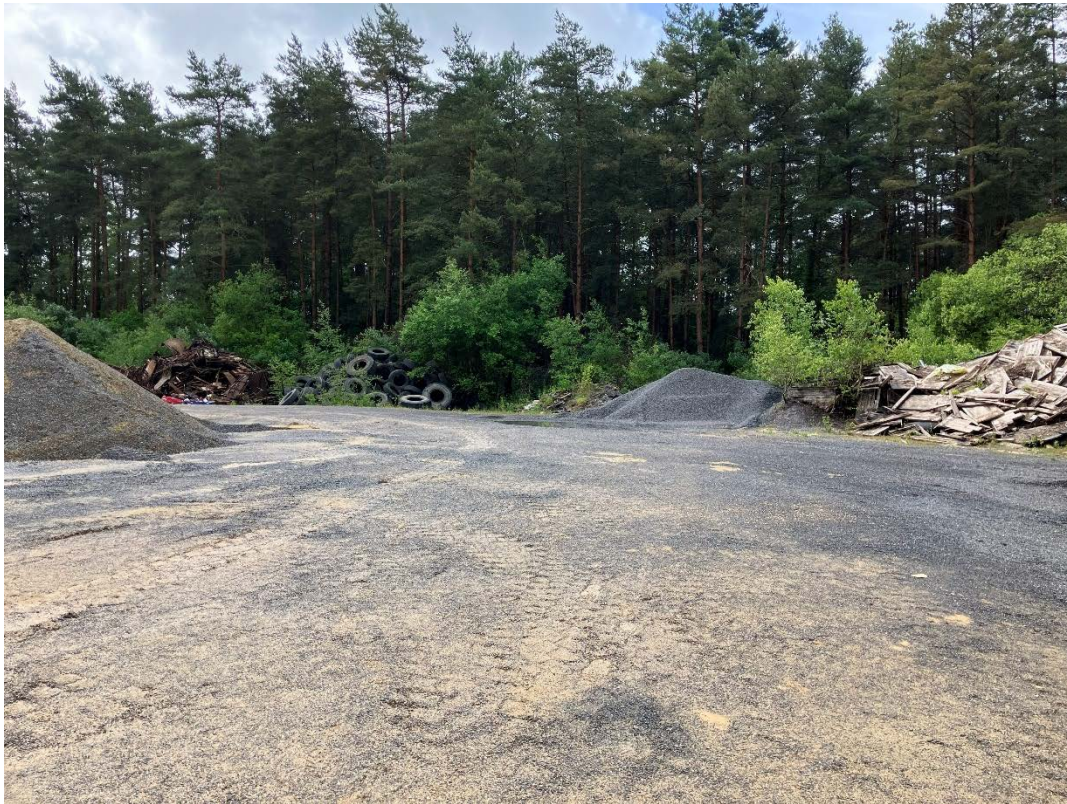
Photograph 23: Materials storage area in south of site – stockpiles of raw materials, pallets, scrap metal and used tyres. Looking southeast.
