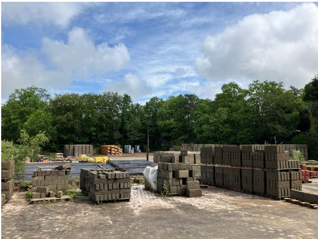
Photograph 6: Site overview – storage of blocks. Looking east.
