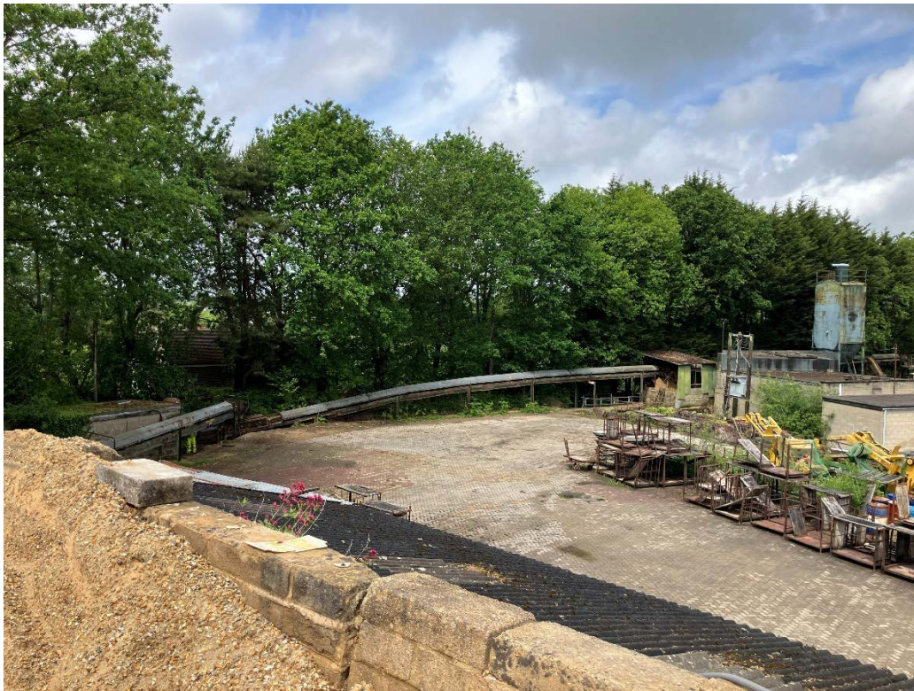
Photograph 26: Overview of conveyer from hoppers of raw materials. Looking northwest.
