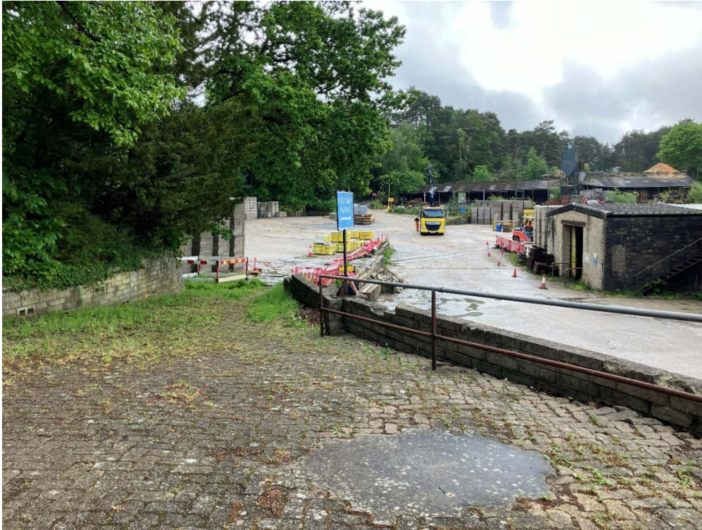
Photograph 1: Overview of yard. Looking south.
