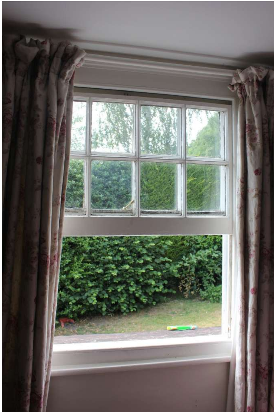
Plate 70. Sliding sash window in the first floor room of the rear outshot.
