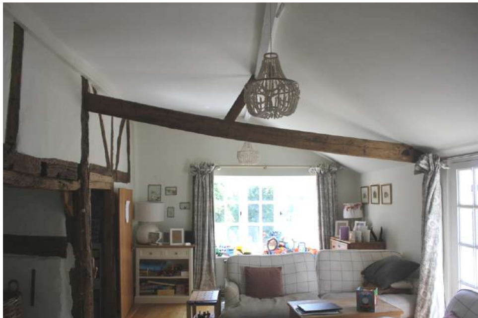
Plate 73. Roof tie of the single storey structure.
