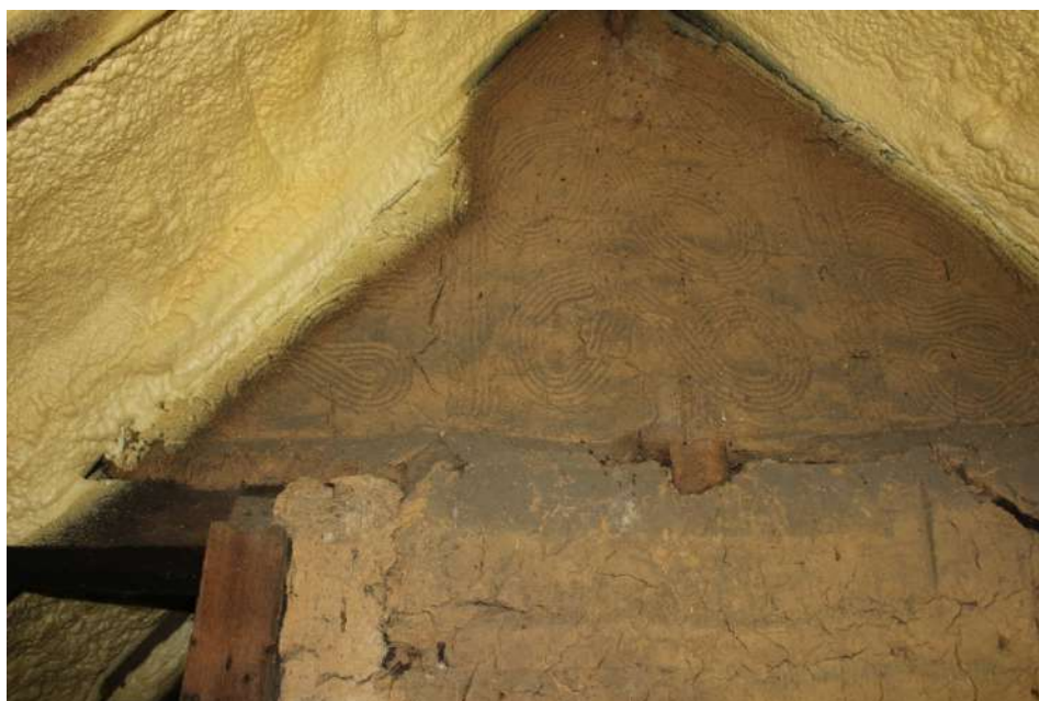
Plate 25. Partitioning of the open Truss C (clean stud to the left is from a later period)
