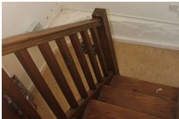
Plate 89. Modern steps leading to the lower basement level.
