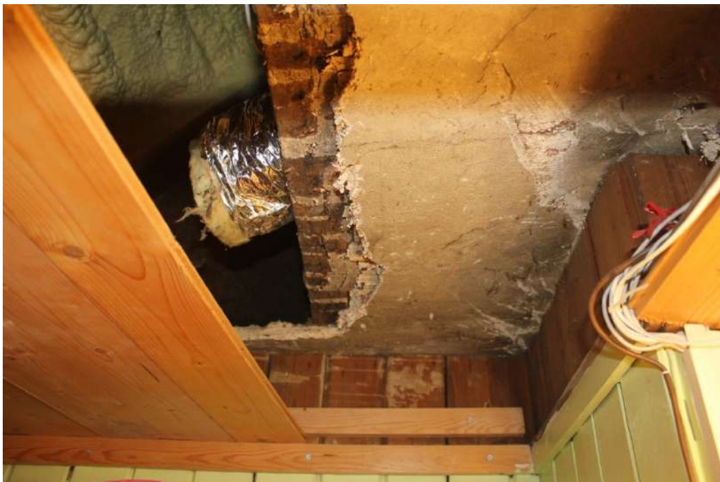
Plate 60. Period D lime plastered ceiling exposed in the cupboard space on the west side of the chimney stack.
