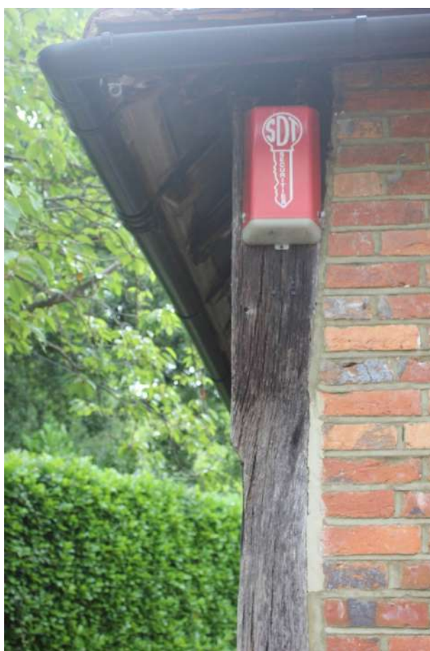
Plate 20. Un-conventional re-use of a post with out-turned jowl.
