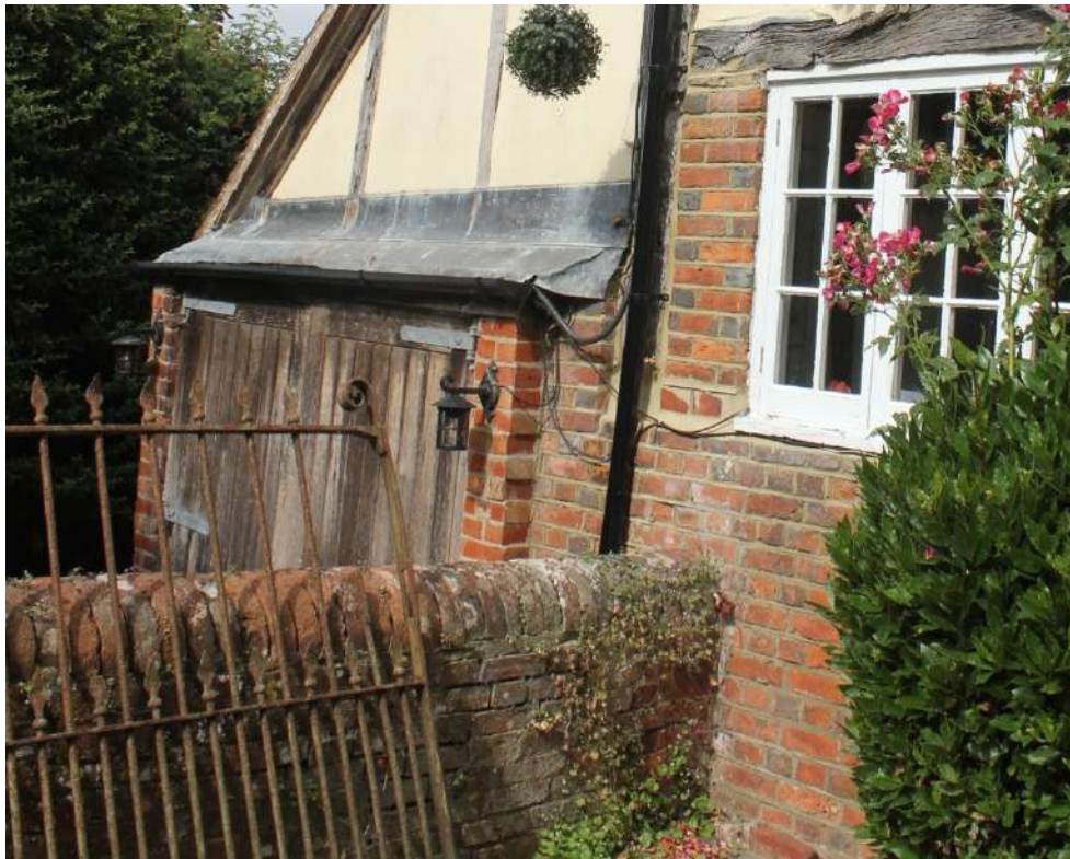
Plate 55. Brickwork in the east elevation of the house extends across the front of the outshot although there are later projecting piers.
