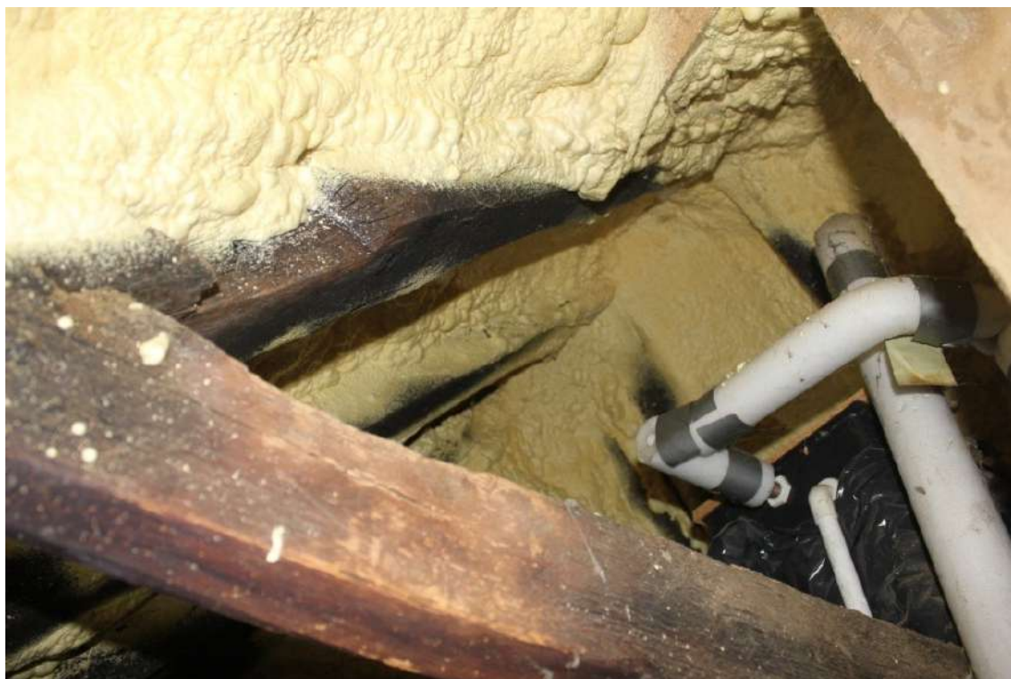
Plate 30. Later collars attached to sooted rafters in Bay 1.
