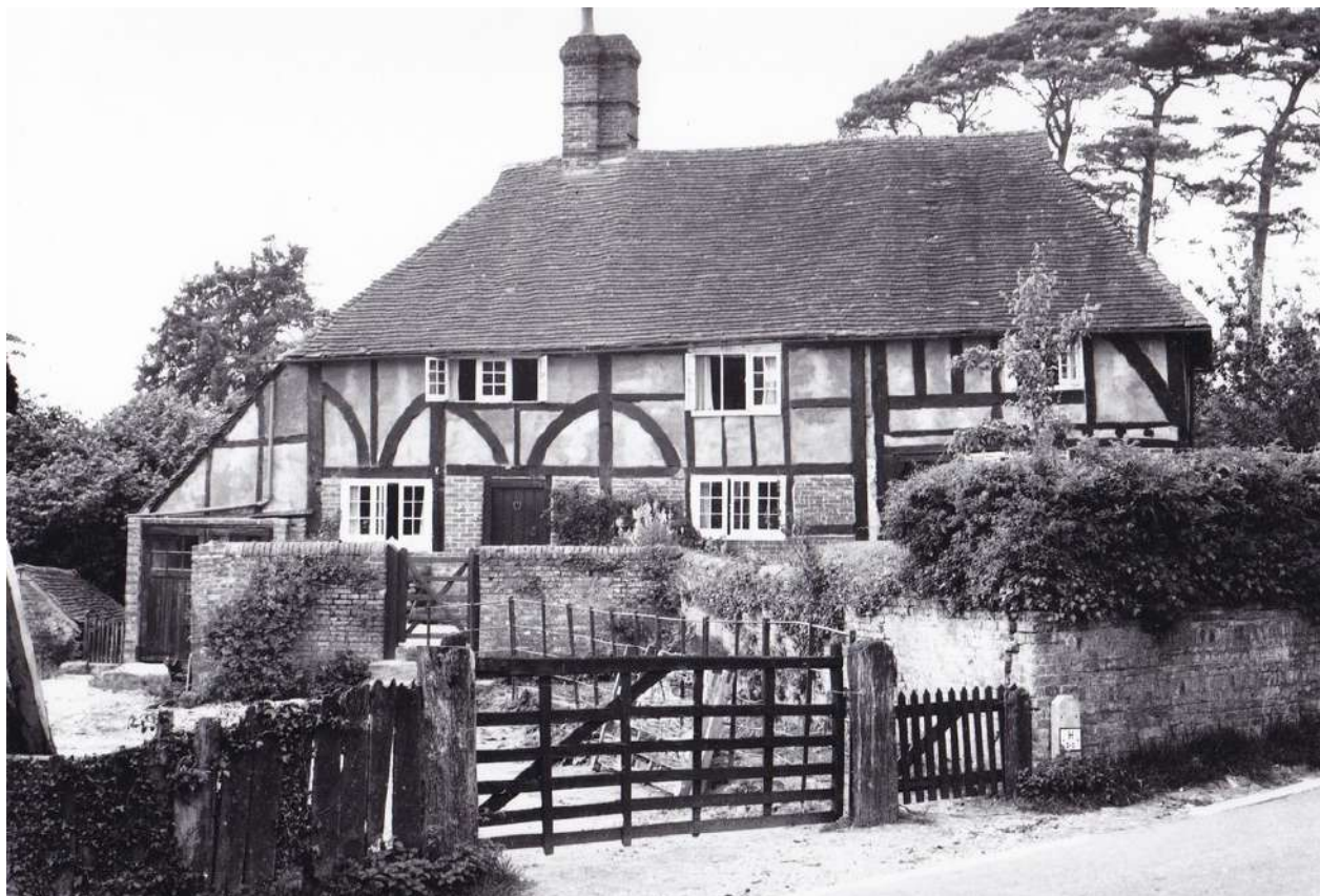
Plate 2. Photograph of the front of the Farmhouse after the removal of the tile hanging in 1965.
