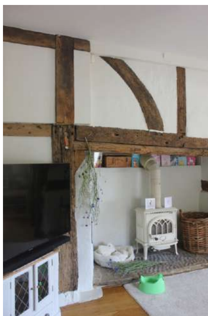
Plate 90. False hearth created for the log burner.
