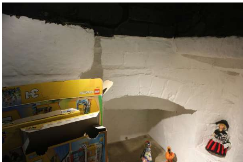
Plate 64. Segmental arched bread oven lintel to the side of the fireplace in Bay 2.
