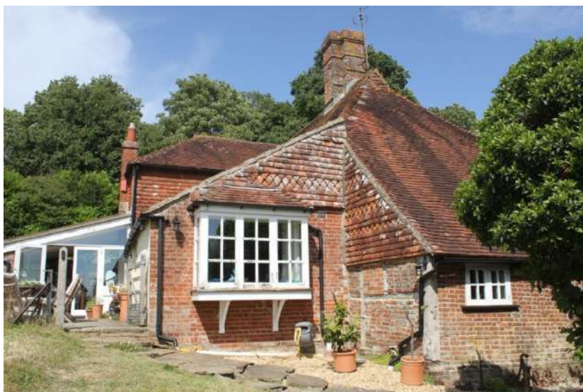
Plate 81. Modern bay window in the south wall of the rear outshot.
