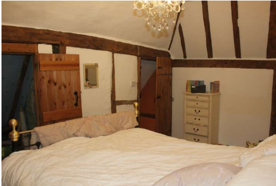
Plate 57. First floor door inserted in the west side of Truss A.
