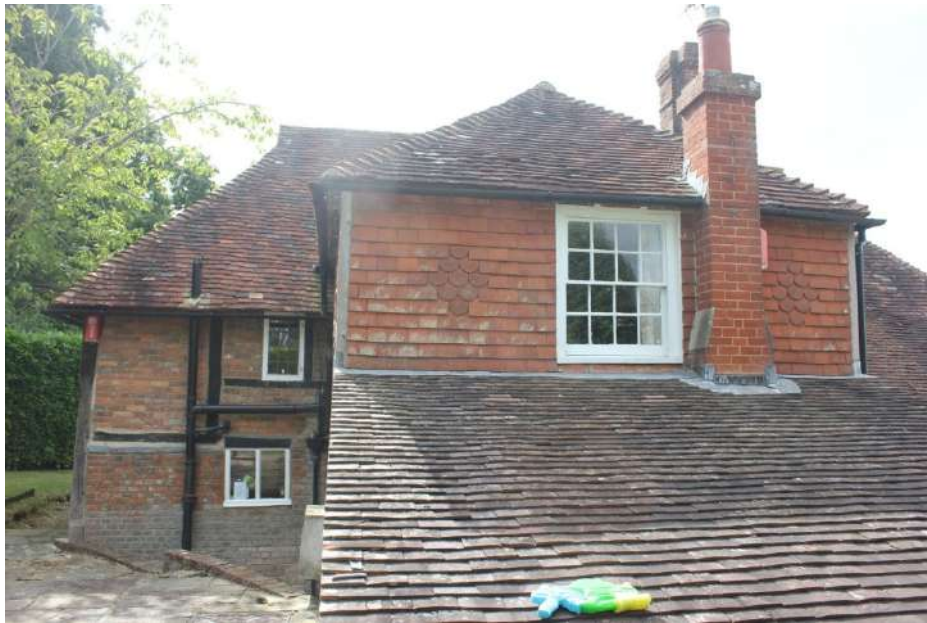
Plate 68. Possible two-storey later extended outshot which is timber-framed.
