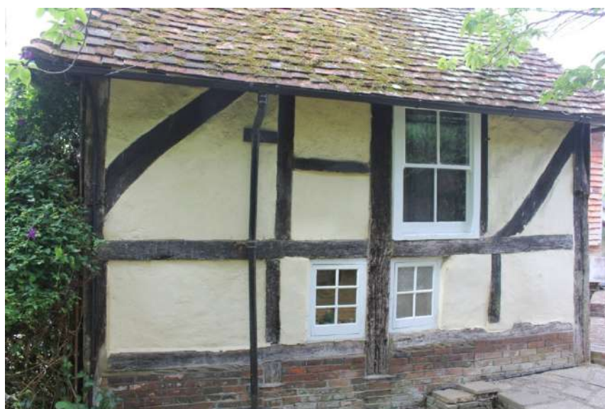
Plate 24. The north side of the cross range with central bay post with mis-matched braces.
