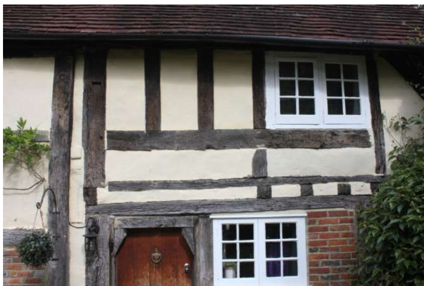
Plate 21. The east side of the Period B cross wing with later timbers nailed into place.
