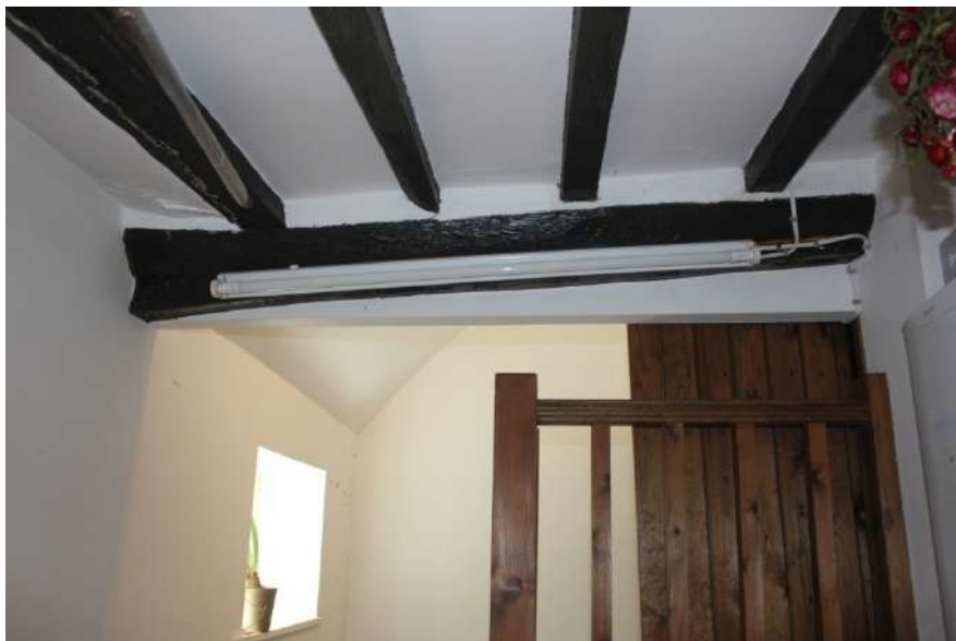
Plate 58. Slim joists used in the lower outshot ceiling.
