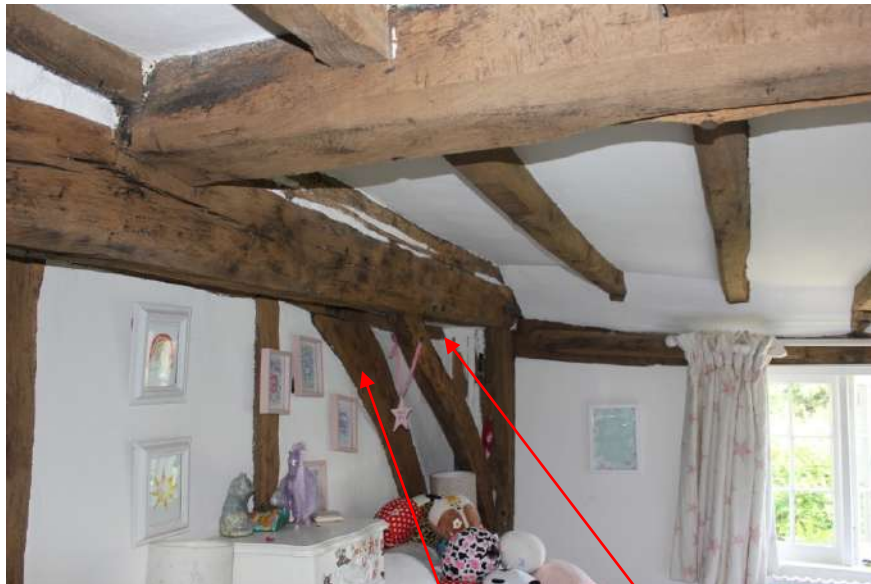
Plate 8. Two frames evident where the inserted Truss D meets the braced wallplate of the Period B attachment.
