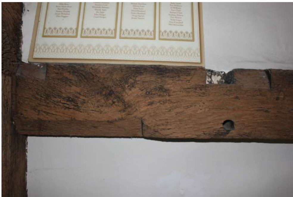
Plate 21. Chamfered southern wall plate of the Period B cross wing with empty birds mouth rafter scotch.
