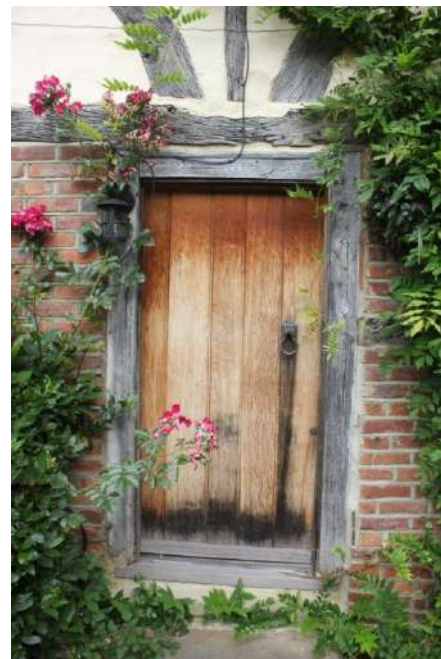
Plate 83. Northern entrance door to east.
