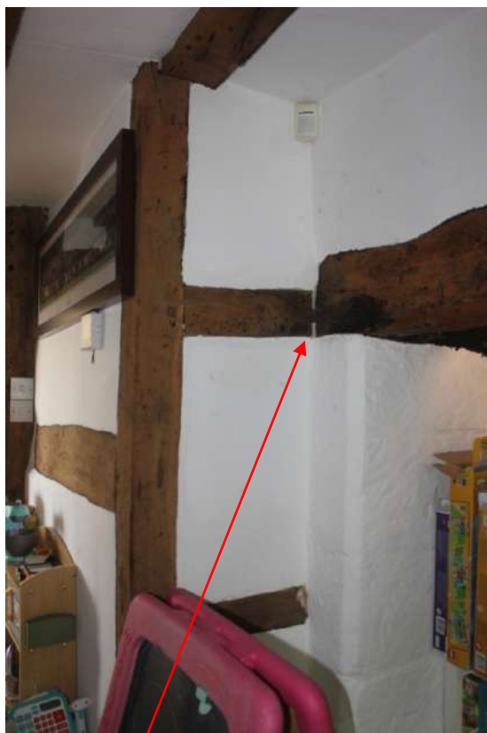
Plate 45. Partition wall morticed to the stack wall creating the side of the stairwell.
