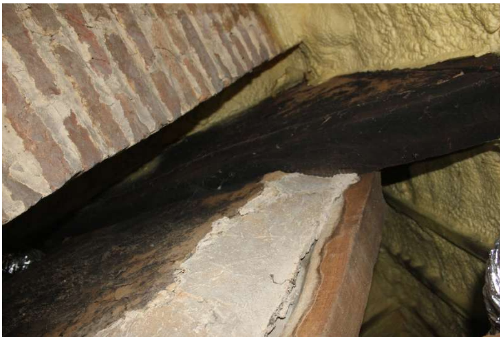
Plate 34. Inserted doorway in the roof space in Truss C and daub repairs.
