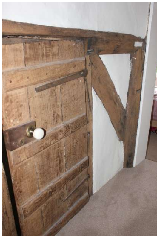
Plate 36. Low door in the western side of Truss D.
