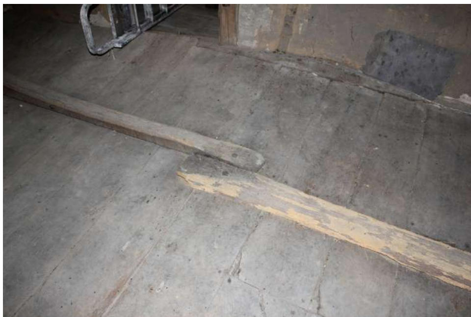
Plate 41. Period C floorboards in-situ in the roof space of Bay 3.
