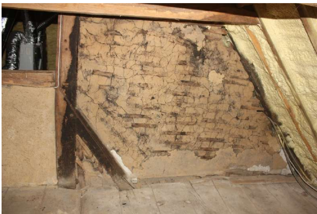
Plate 32. South side of the crown post which is soot stained but with later daub applied to the panel.
