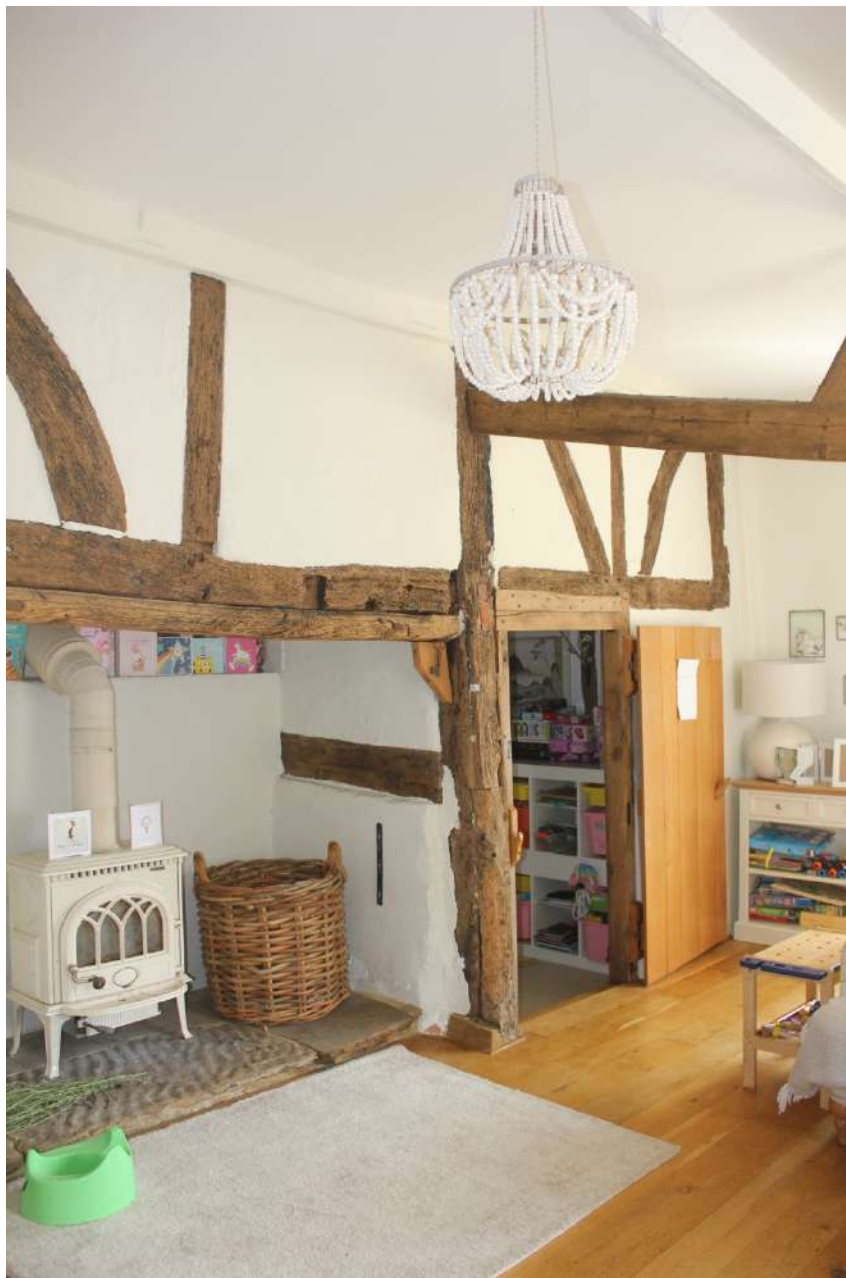
Plate 71. New Period E doorway created in the west wall of Bay 1.
