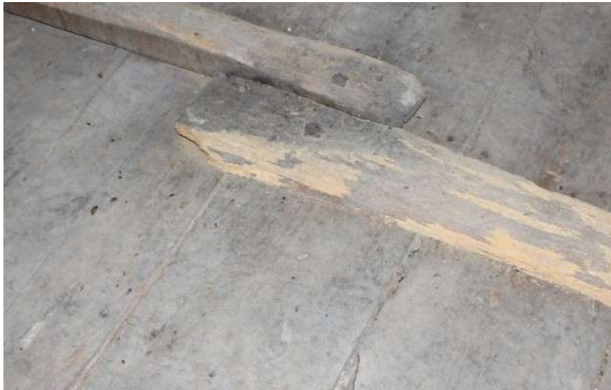
Plate 61. Large retaining beams bolted to the Bay 3 boards in the attic.
