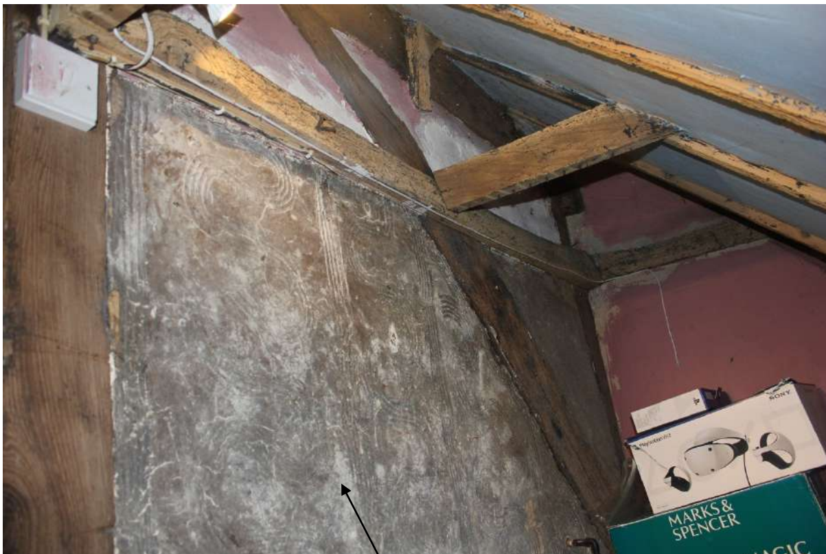
Plate 5. Comb decorated daub under the paintwork in the south side of Truss A.
