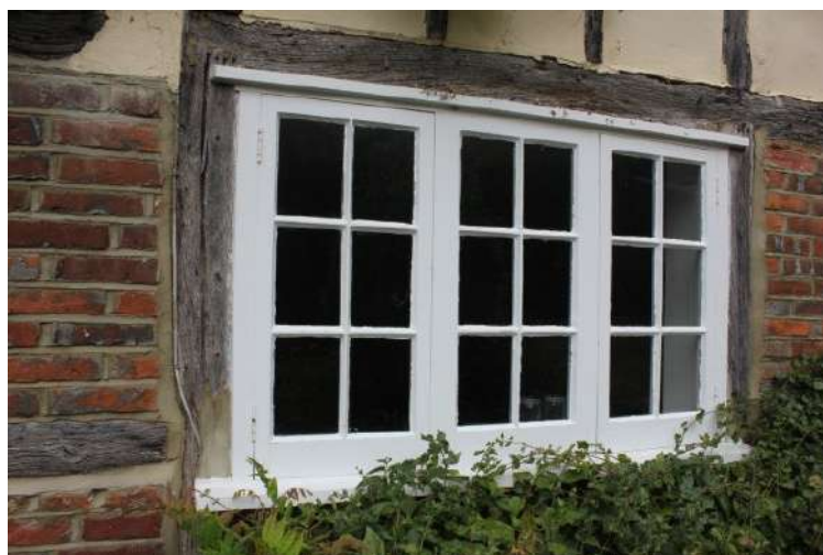
Plate 78. Modern casement window in the east elevation of Bay 3.
