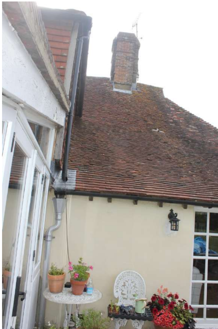
Plate 69. Rendered rear wall of the outshot with catslide roof.
