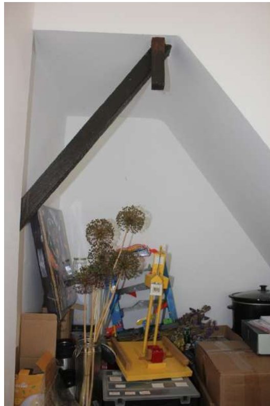
Plate 65. Slim roof ties in the outshot.
