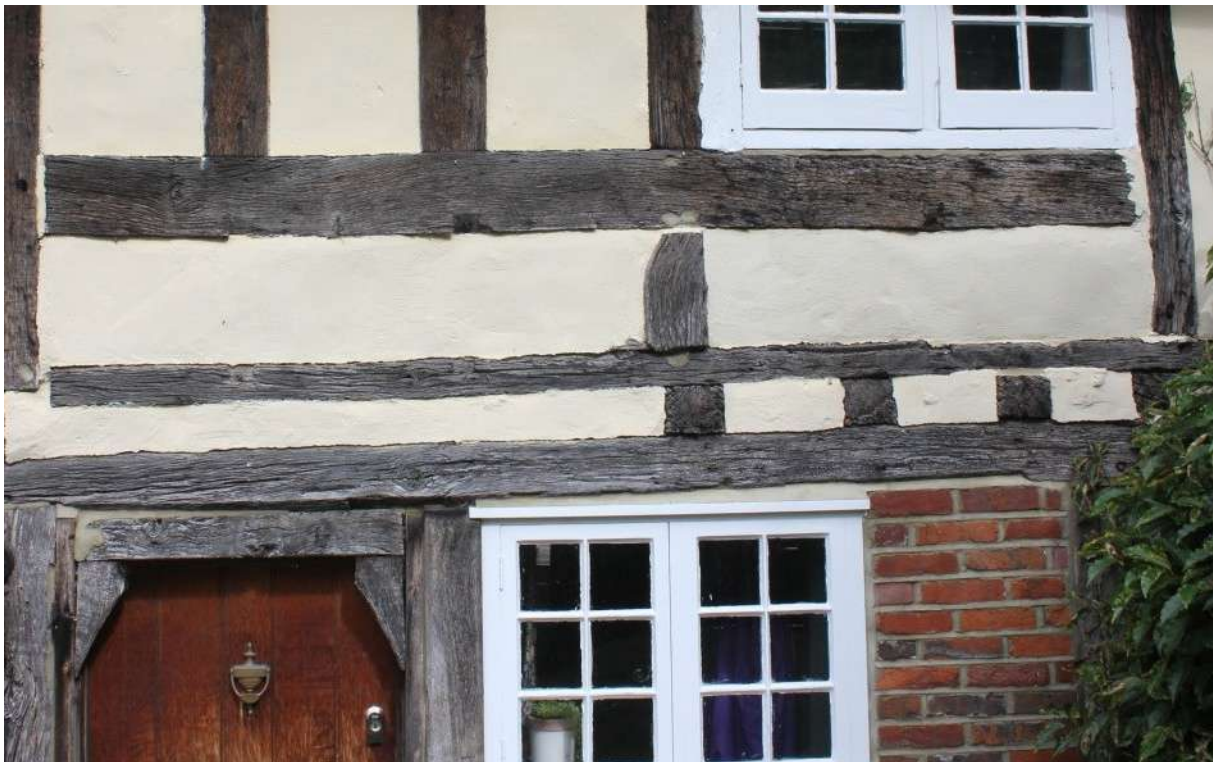
Plate 27. Exposed floor joists over half the width of the range which cannot be interpreted.
