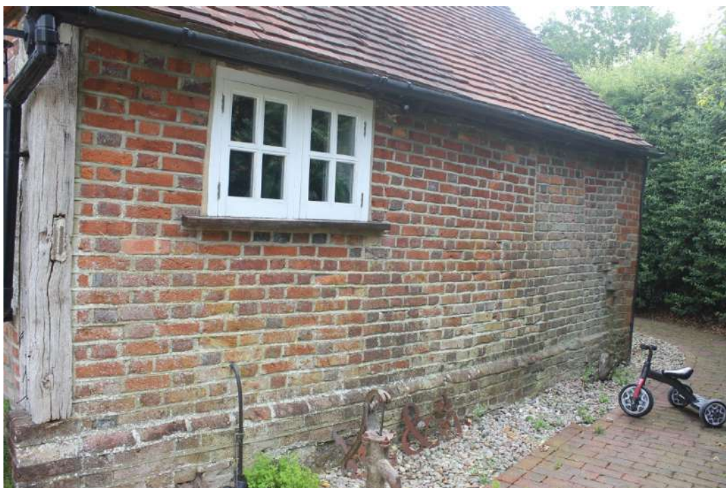
Plate 56. Blocked Period D window in the south wall of the outshot.
