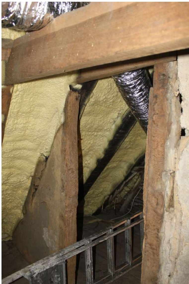
Plate 37. North side of the Period C doorway created in Truss C to the east.
