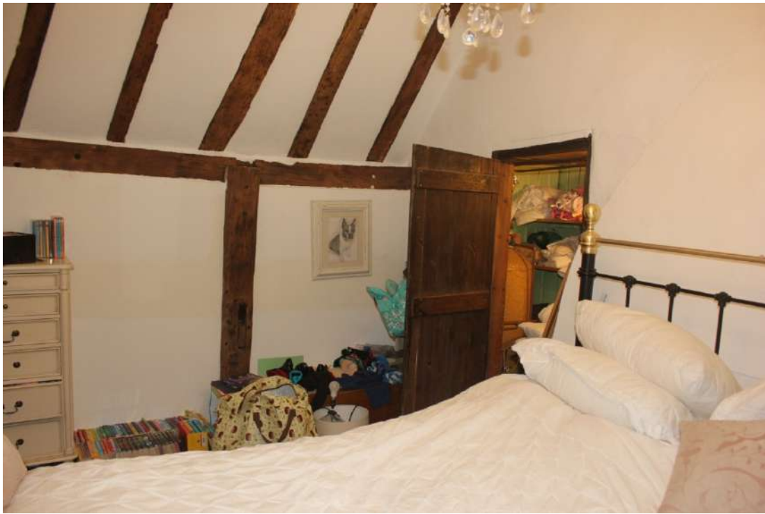
Plate 59. Raised ceiling height in the first floor chamber of Bay 1.
