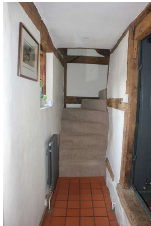
Plate 88. Modern tiles in Bay 5 corridor.
