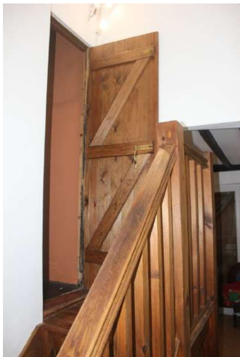
Plate 84. Door of the lower southern outshot.
