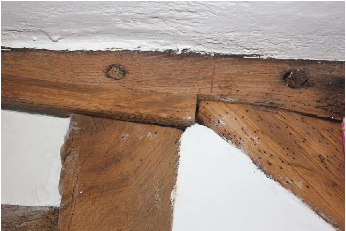
Plate 51. Inserted brace cut into the Truss C tiebeam.
