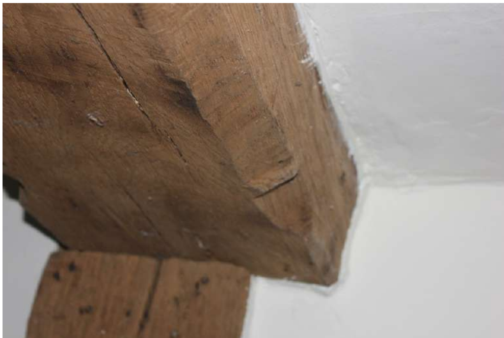
Plate 40. Bar and curved stop chamfer decoration on the central girder in Bay 3.
