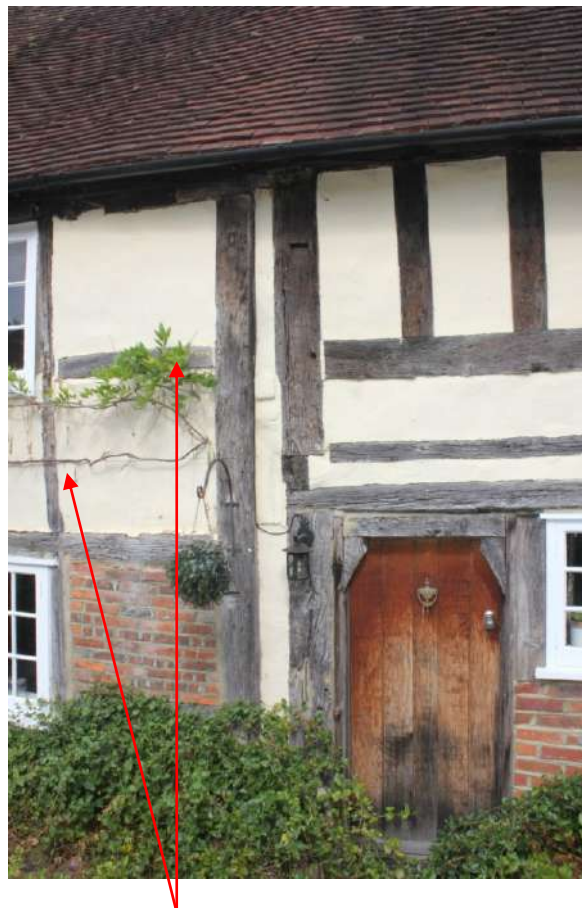
Plate 9. Re-set timbers infilling the former hall window to the east.
