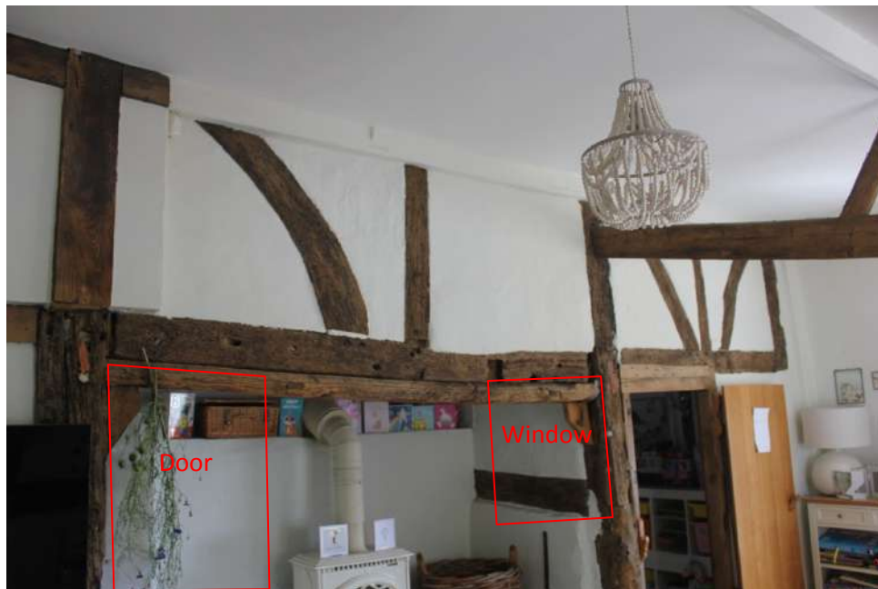
Plate 11. The west side of Bay 2 with removed features outlined in red.
