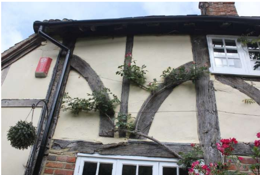
Plate 3. The steeply curved braces in the east side of Bay 1.
