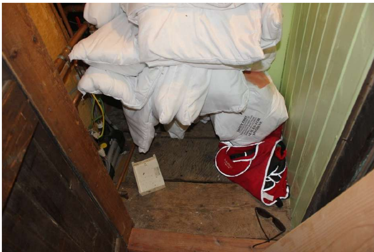
Plate 42. Glimpse of Period C floorboards in the cupboard to the west side in Bay 2.
