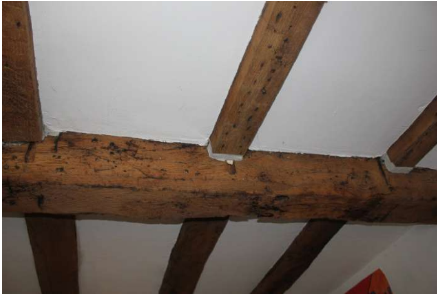
Plate 38. Inserted girding beam and joists in Bay 1.
