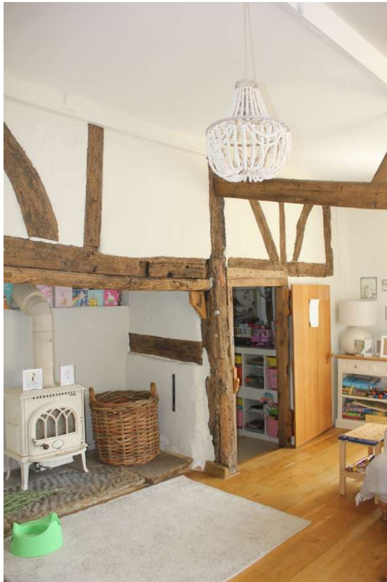
Plate 43. Location of the former stairs within the modern fireplace aperture.
