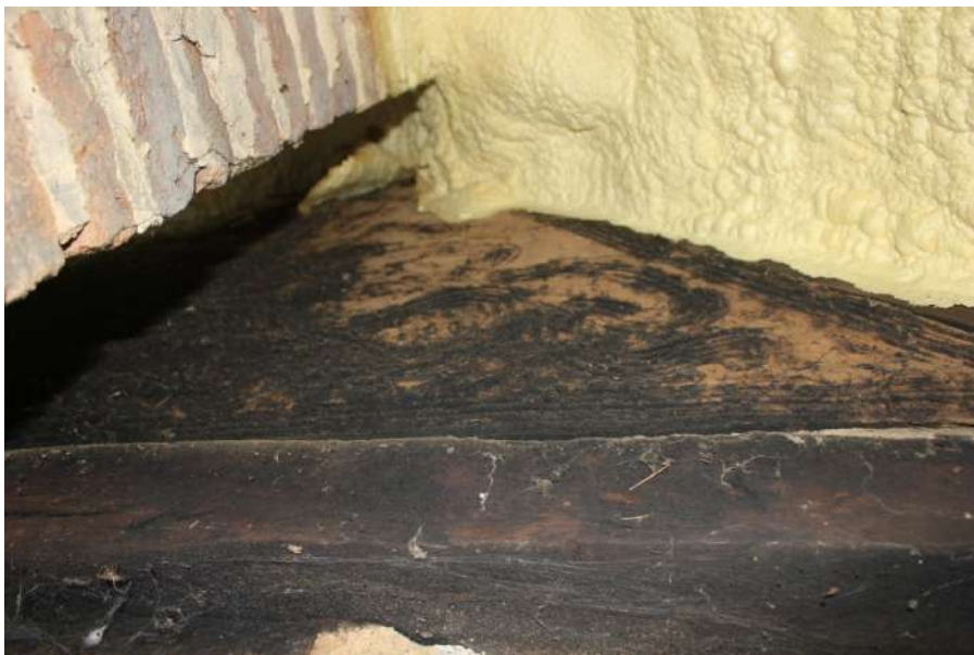
Plate 16. Later sooted infill panel above the collar in the open Truss C.
