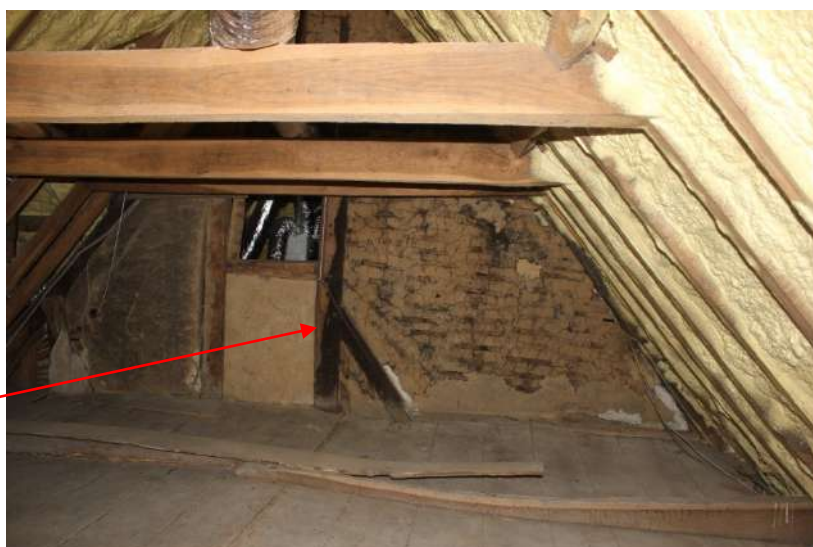
Plate 17. Period D roof replacement in Bay 3 only, which is not soot stained.
