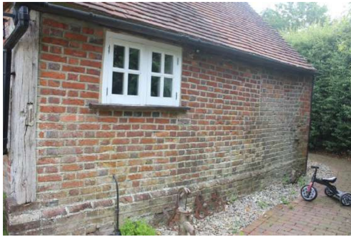
Plate 79. Four light casements in the south wall of the southern outshot.
