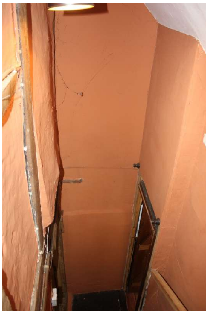
Plate 52. Lath and plaster internal walls in the outshot.
