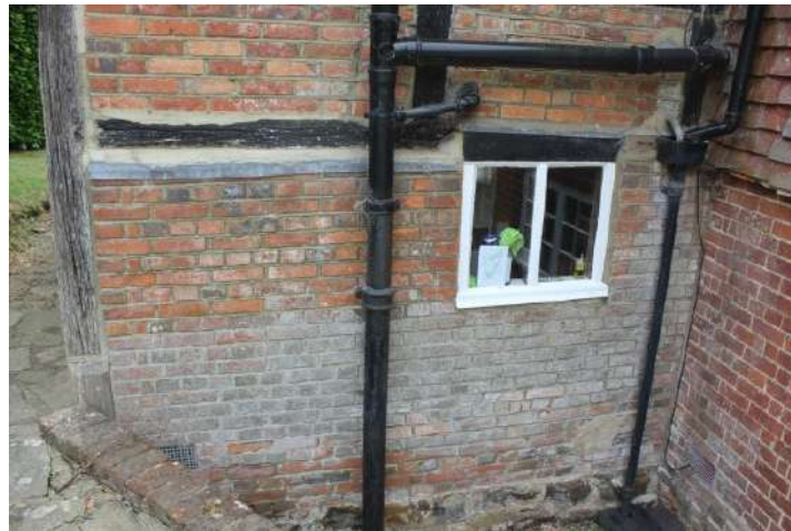
Plate 80. Two light casement in the west side of bay 5.
