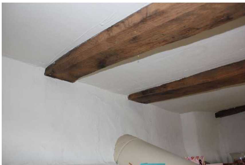
Plate 44. Inserted joists for the stair landing inside the modern fireplace aperture.
