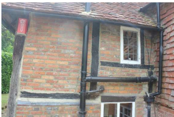
Plate 26. Presence of a pegged stud and window cill in the west side wall of the cross range.
