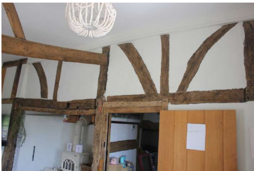
Plate 4. The curved bracing the west side of Bay 1.
