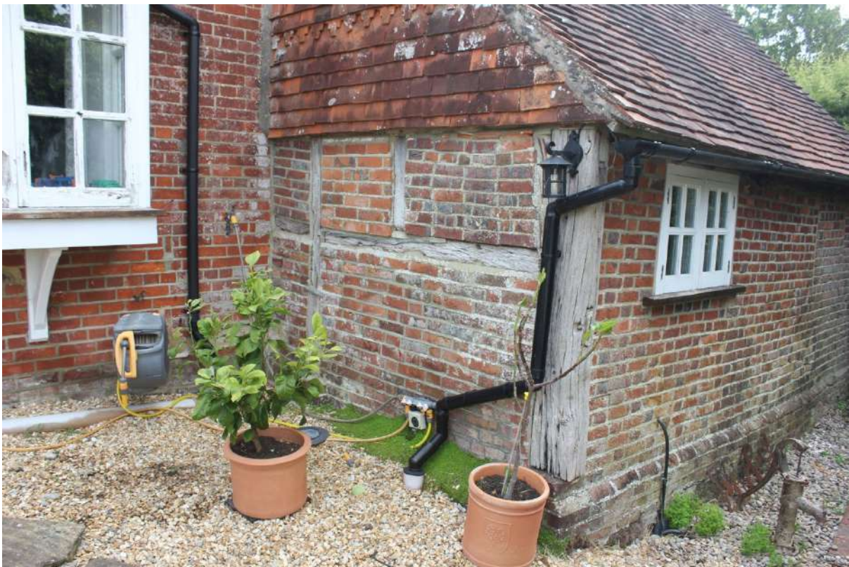
Plate 54. Brick and timber rear wall of the southern outshot.
