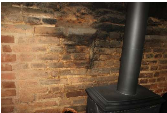
Plate 46. Thin, Tudor bricks within the hearth serving the Bay 3 parlour.
