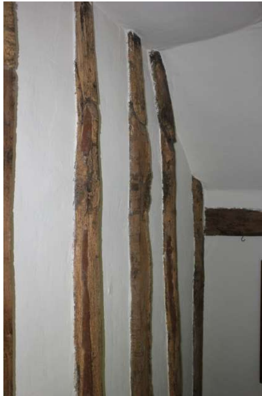
Plate 77. Re-used timber in the north wall of the first floor washroom.
