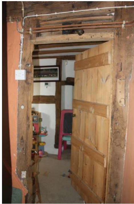
Plate 35. Period C doorway created in the Period A2 Truss A at ground floor level.
