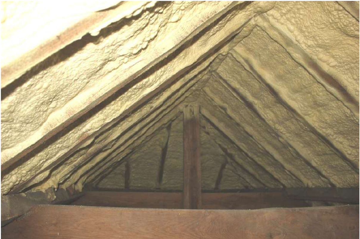
Plate 74. Slim, softwood rafters present in the rear outshot roof.
