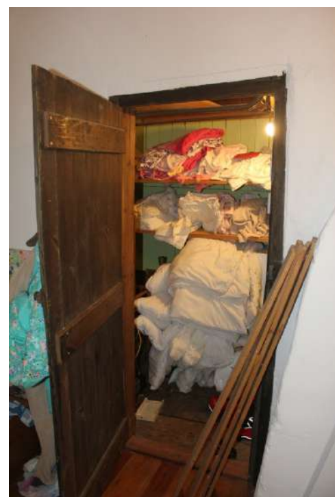
Plate 85. First floor door west of the stack.
