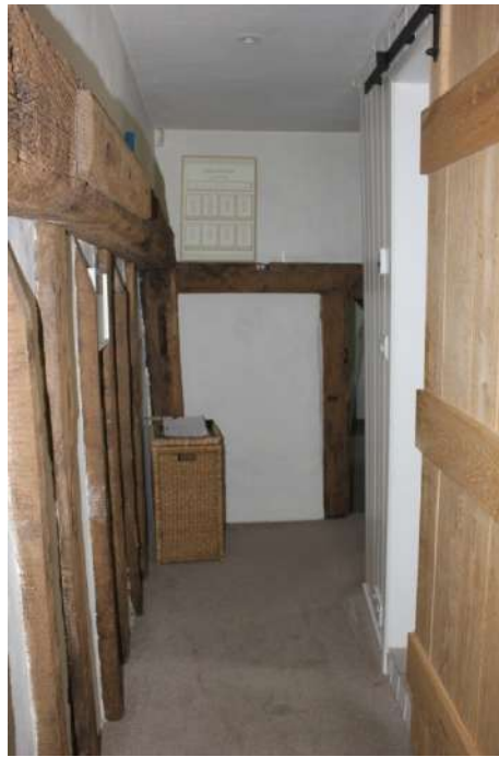
Plate 86. New sliding door in the first floor washroom of Bay 5.
