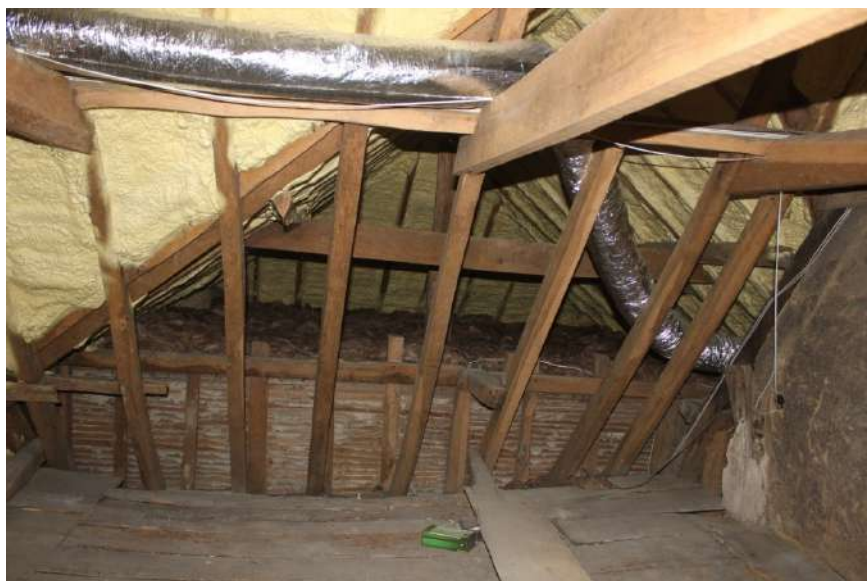
Plate 66. New rafters, collars and side purlin of the Period D roof in Bay 3.
