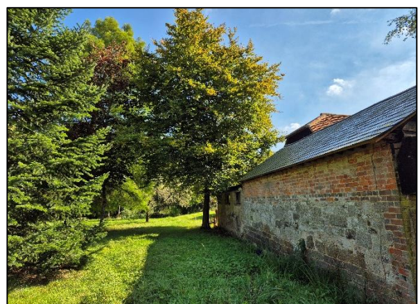
Photo 18: Barn 3 north elevation.
