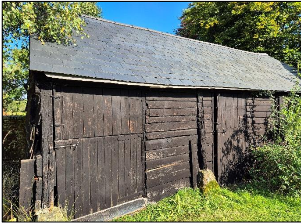
Photo 19: Barn 3 south elevation.
