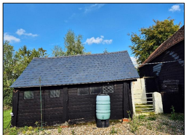
Photo 22: Barn 4 south elevation.
