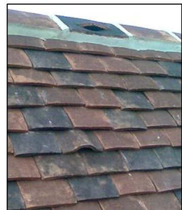
Figure 6.1 Bat access roof tile and ridge tile.
