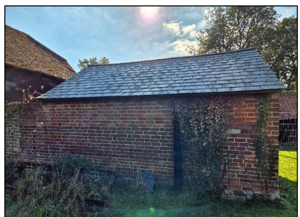
Photo 24: Barn 4 north elevation.
