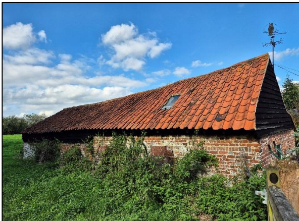
Photo 15: Barn 2 south elevation.
