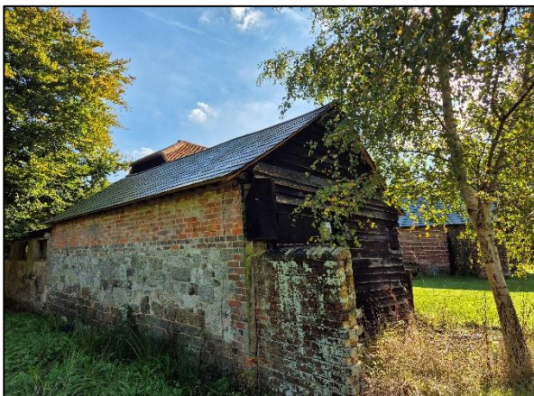
Photo 17: Barn 3 west gable.
