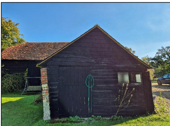
Photo 23: Barn 4 west gable.
