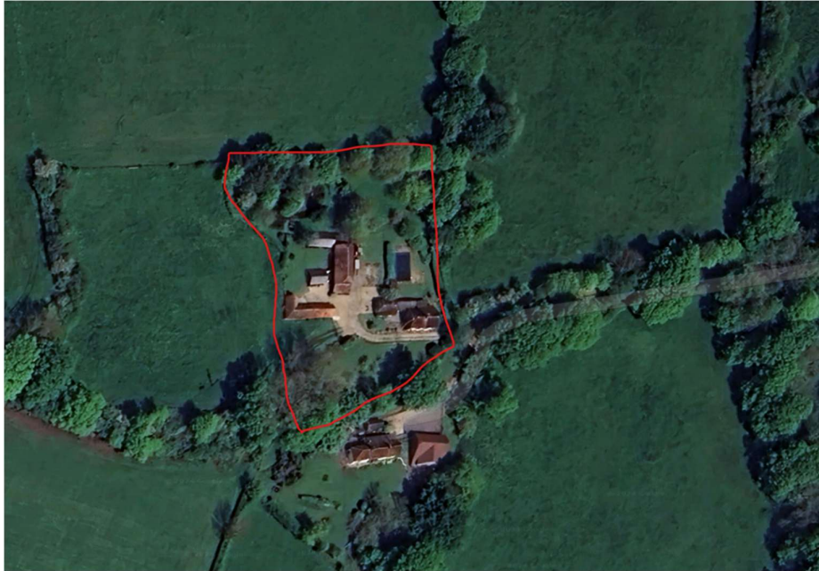
Ariel View of the site (Google)
