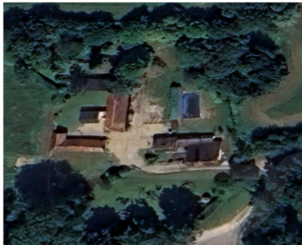
Ariel View of the site (Google)
