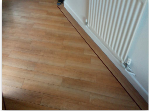
Fig 7.2: Location of buried manhole
