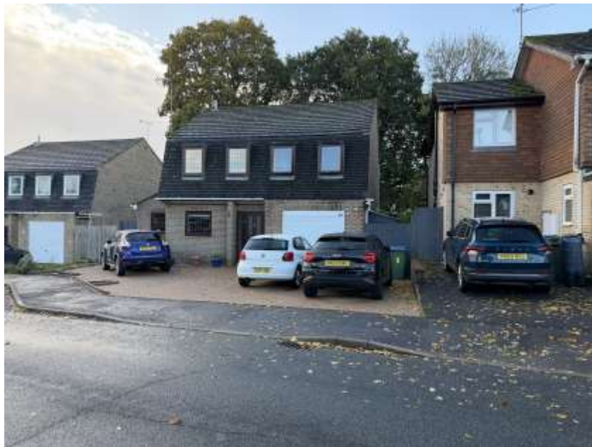
Fig 1. Front elevation of property.
