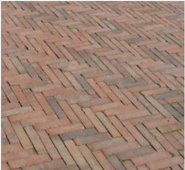
Hurst Quad and Arrival Plaza - Feature paving: Concrete Clay paver look Standard/Non Permeable Build Up
