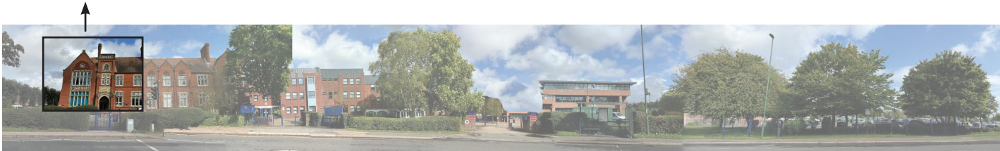
Hurst Road frontage of college buildings & facade articulation of Grammar School Building.
