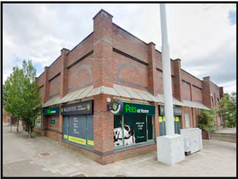
Existing Corner elevation
