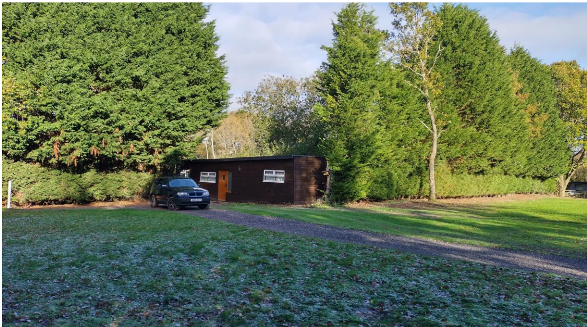
Figure 6: Outbuilding. To be demolished
