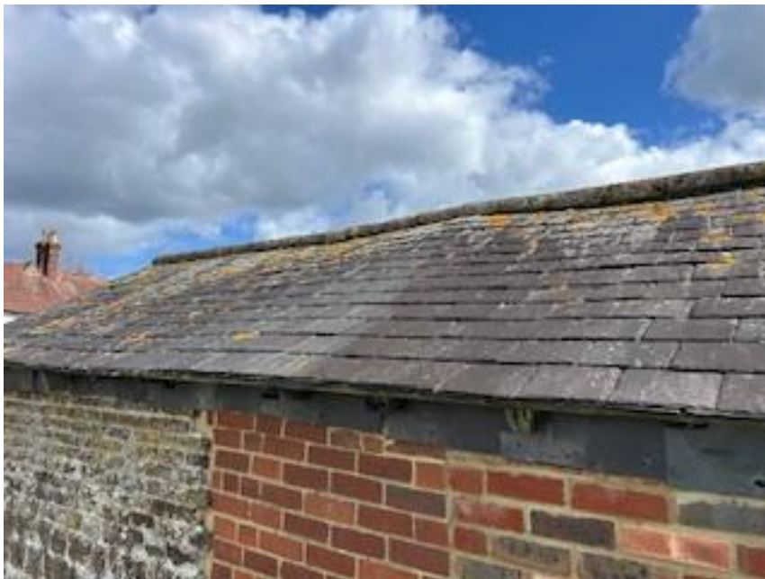
Photo 4 – Detail of B1 roof.
