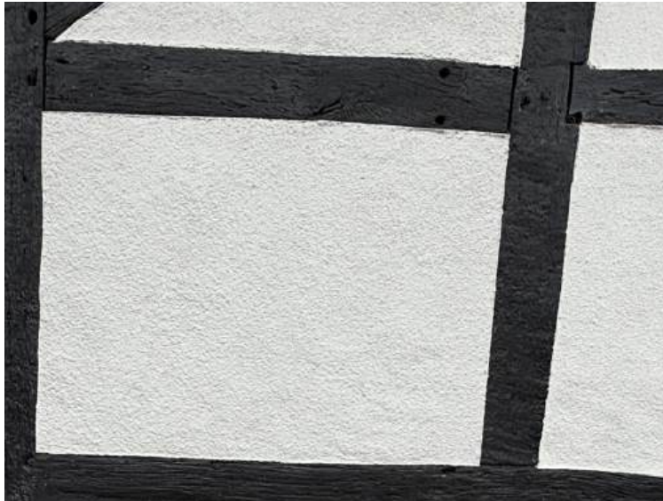
Existing timber framing with render infill to rear elevation
