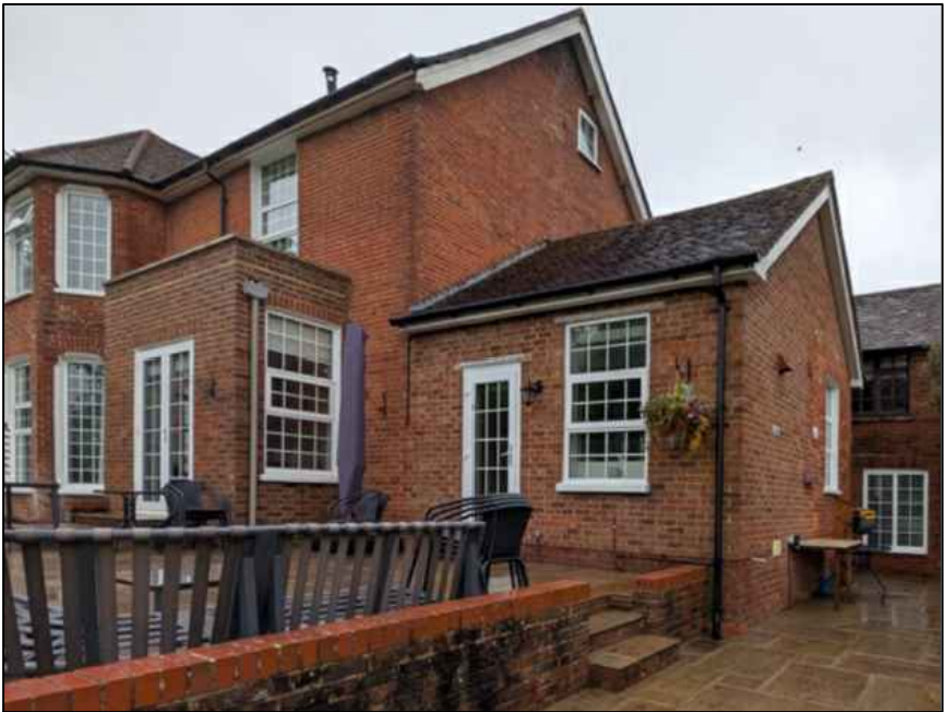
6 - Side (East) View
