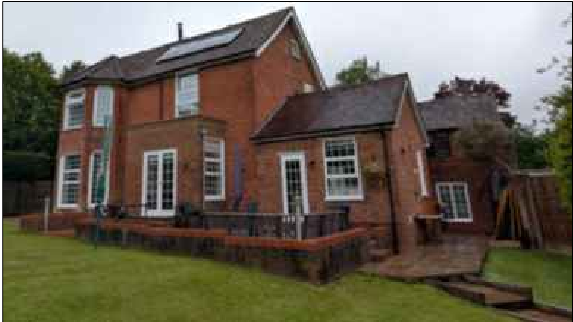
5 - Rear View (South-East Elevation)
