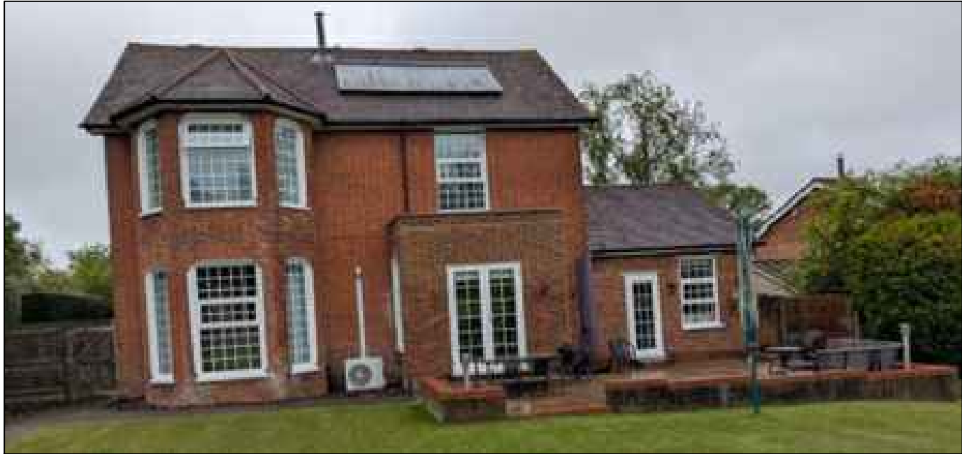
1 - Rear View (South Elevation)
