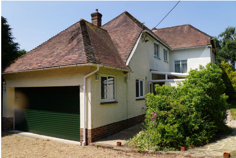
GARAGE TO BE CONVERTED LOOKING WEST
