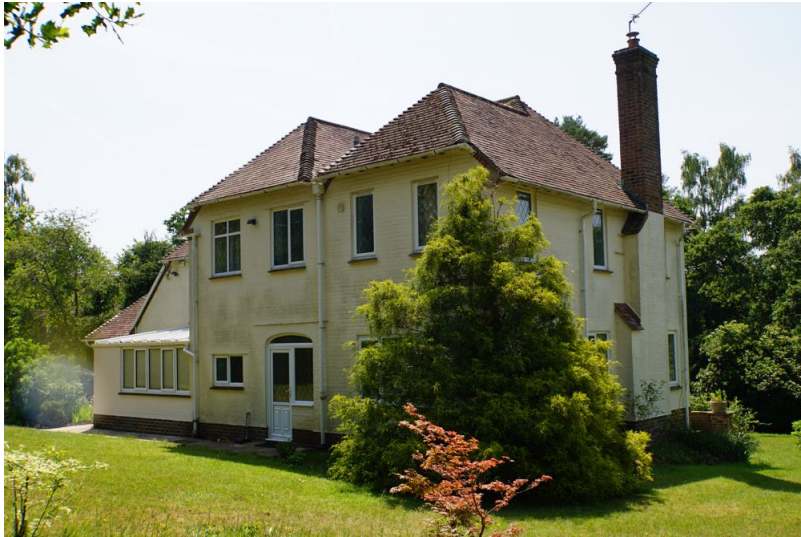
PRINCIPAL ELEVATION LOOKING EAST
