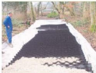
CellWeb during installation.
