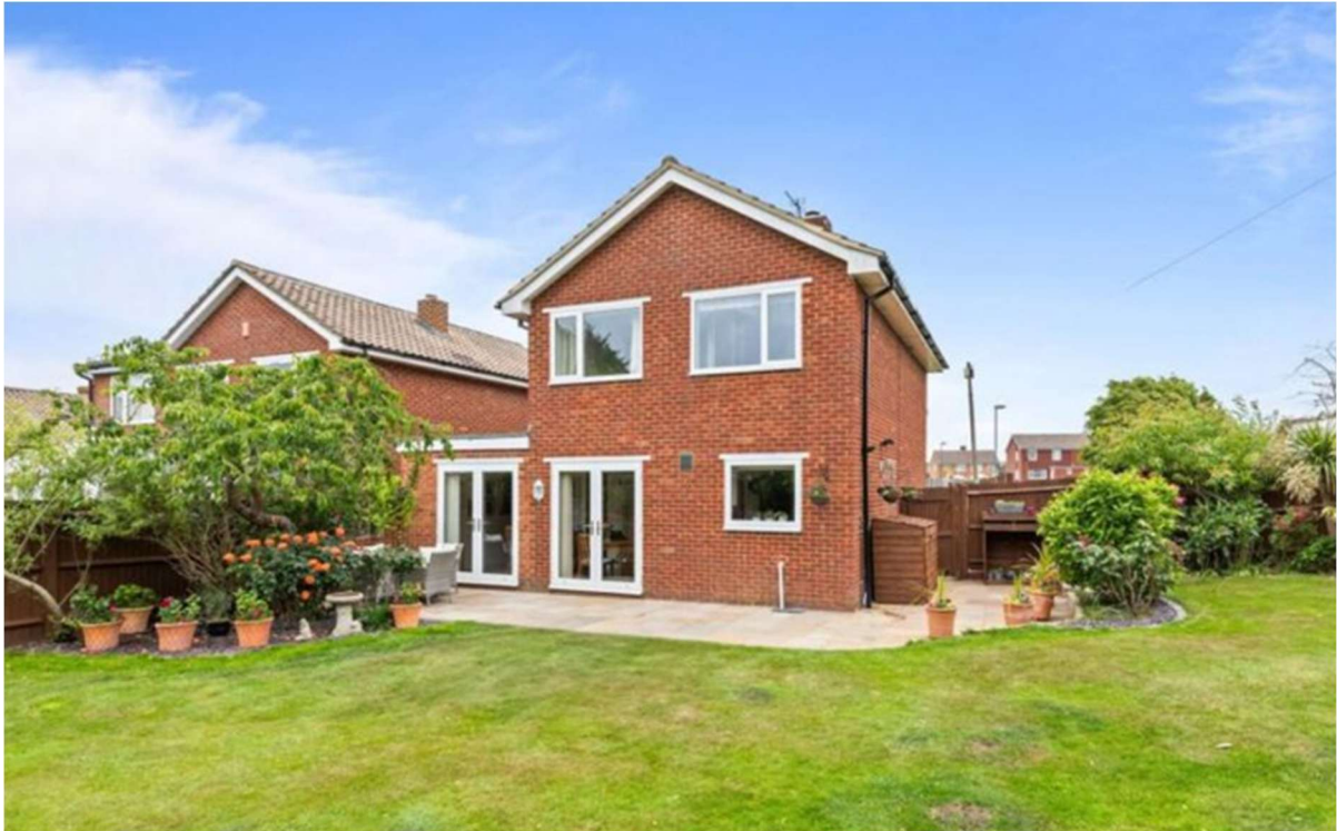
Photo 3: Showing the rear elevation and adjoining property
