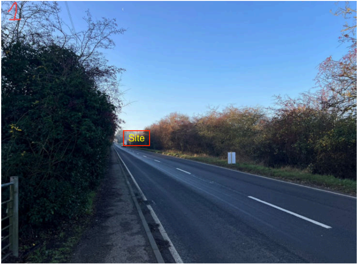
VP1 - A29 Northbound looking south.
