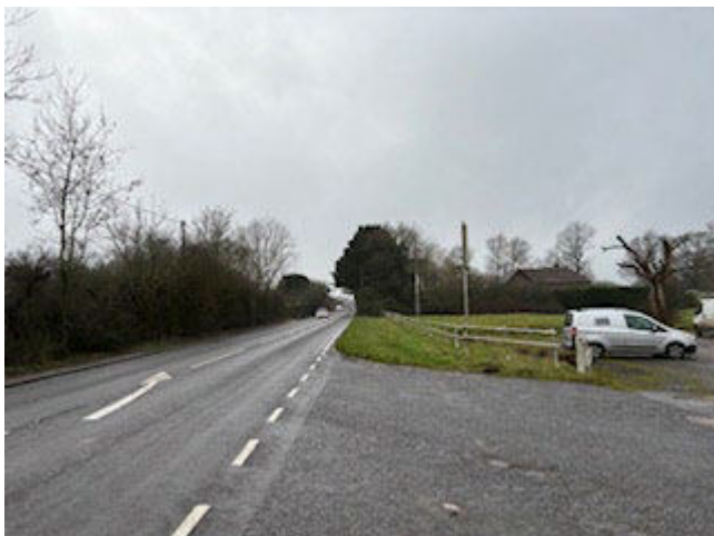
Figure 1: Visibility to the south.
