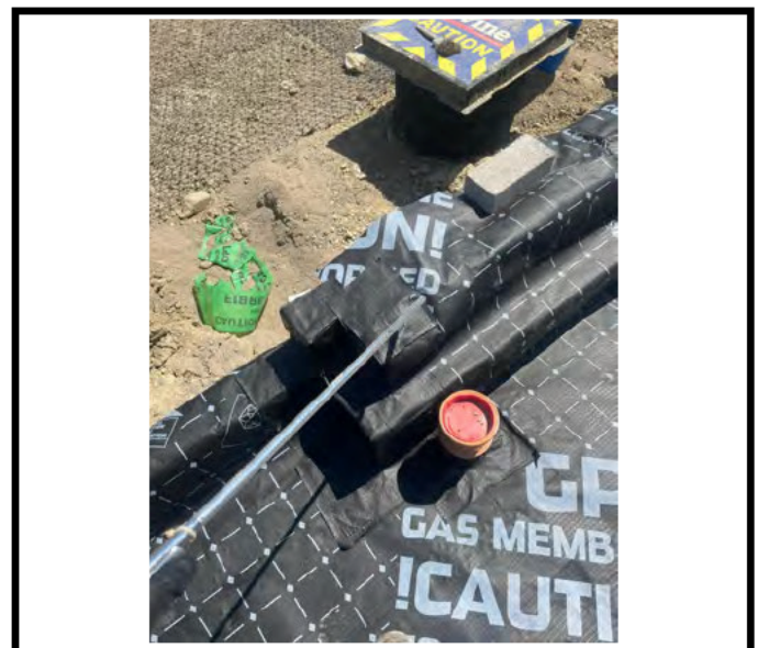
A non destructive air lance integrity test being conducted upon a sealed corner.
