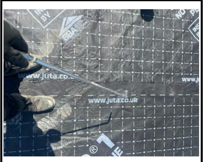
Air lance test on a welded lap.
