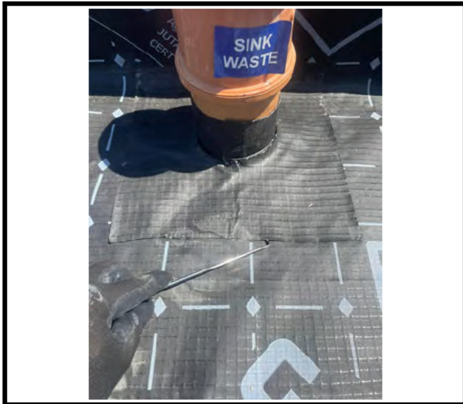
A mechanical point stress test being conducted upon a sealed pipe penetration.
