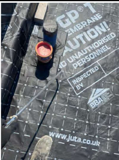
Air lance test on a pipe penetration.
