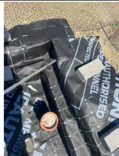
Air lance test on a corner.
