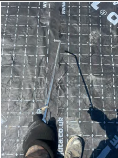
Air lance test on a welded lap.
